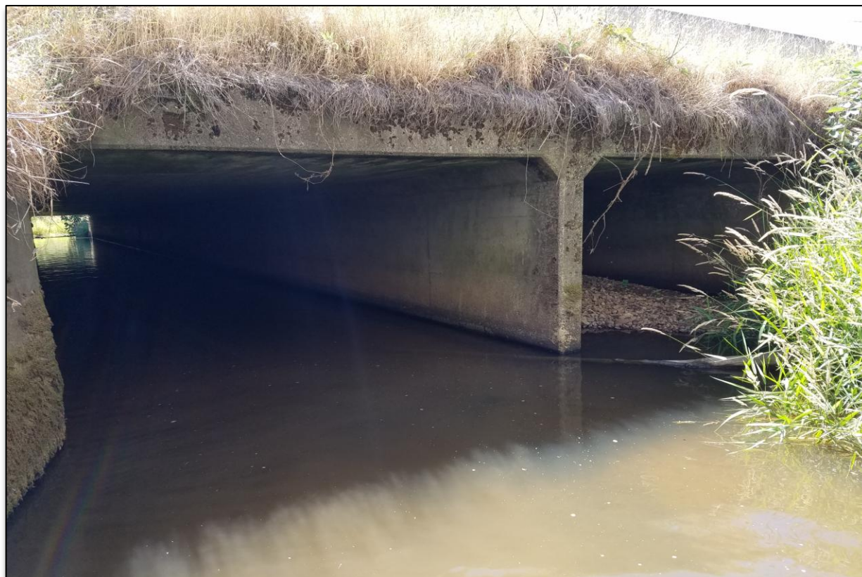
Image 9: DB13: Double Box Culvert under I-5
