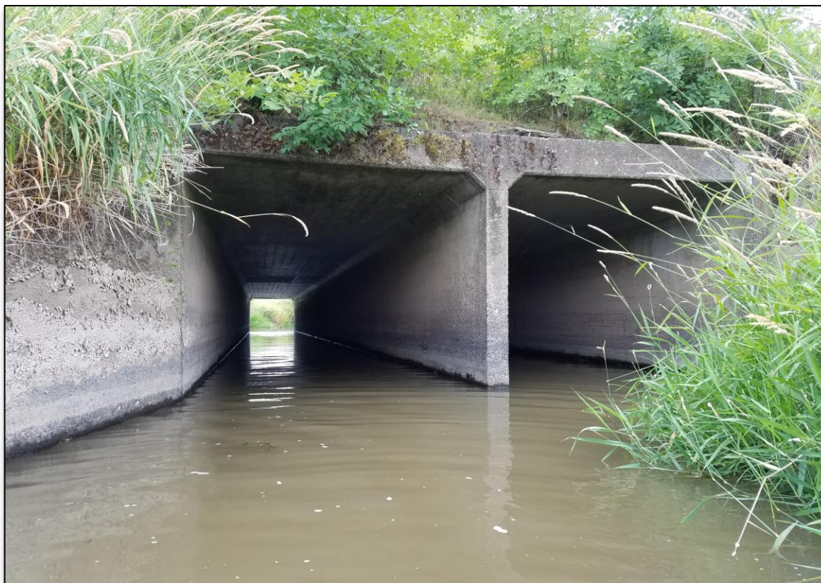
Image 16: DB10: Double Box Culvert under Rice Road
