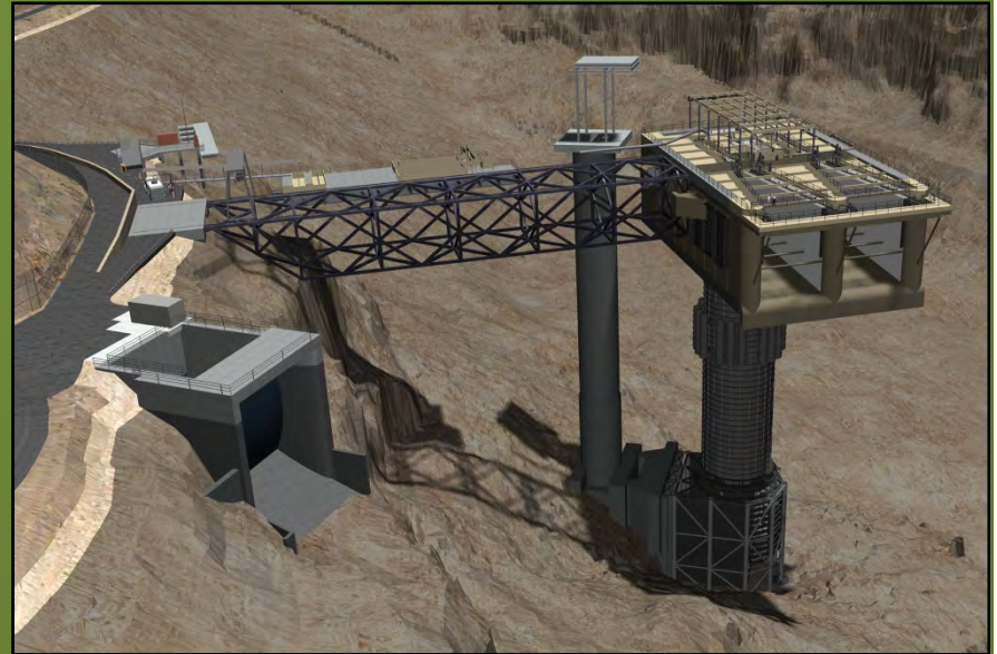
Selective Water Withdrawal Tower and collection facility. Figure by PGE
