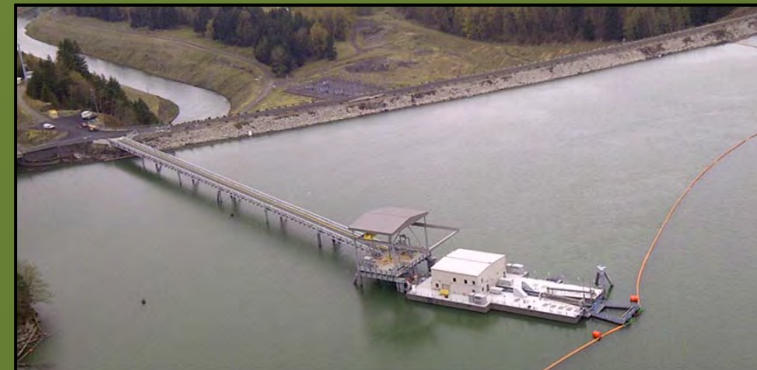
Swift Floating Surface Collector. Photo and Figure from PacifiCorp
