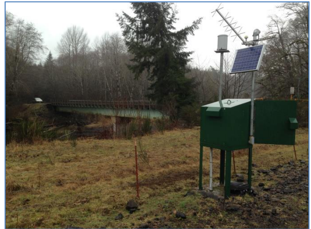
Figure 1: West Fork Satsop Rain Gage (foreground) and New Stream Gage (mounted on bridge in background)
