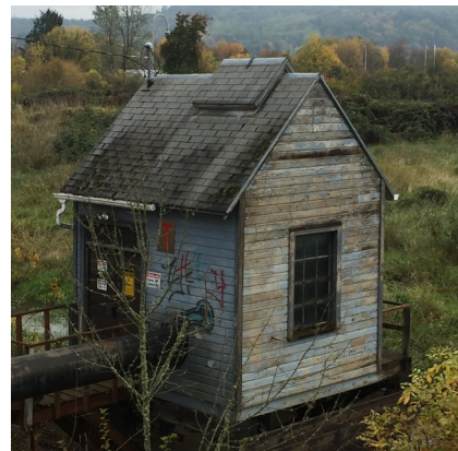
Old Pump – 1940s
