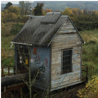
Old Pump – 1940s
