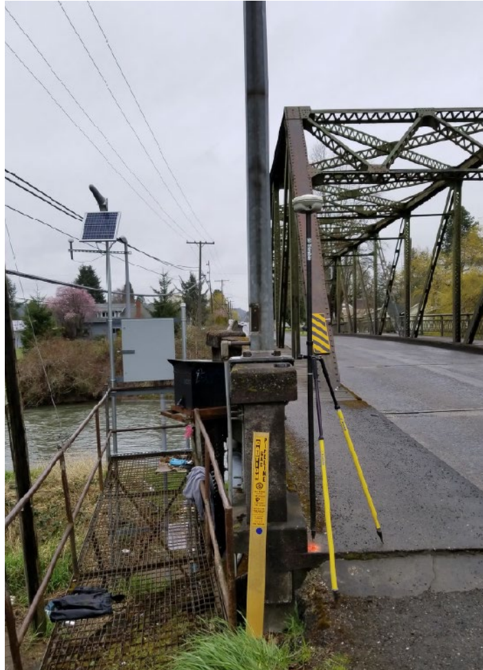
Figure 2.3. Skookumchuck at Centralia being surveyed to NAVD 88. Photo courtesy of USGS.
