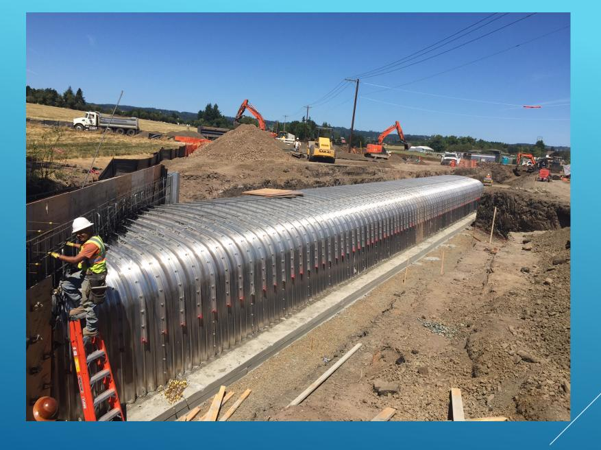
FORMING FOR CONCRETE HEADWALL
