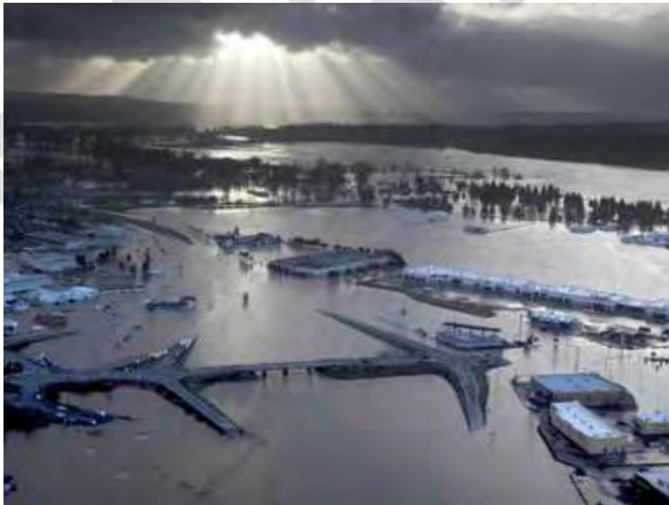
Figure B-1. Image of Flooding During the 2007 Chehalis Flood
