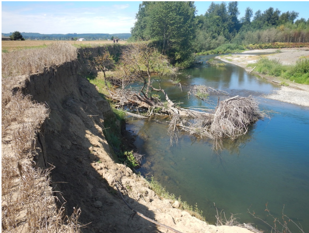
Figure 1. Eroding Bank looking upstream along right-bank of Satsop River, August 2015
