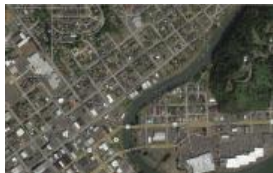
Market Street Dike
