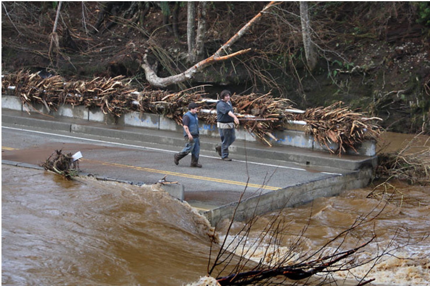
Chandler Road Bridge near Doty, WA STEVE RINGMAN / SEATTLE TIMES
