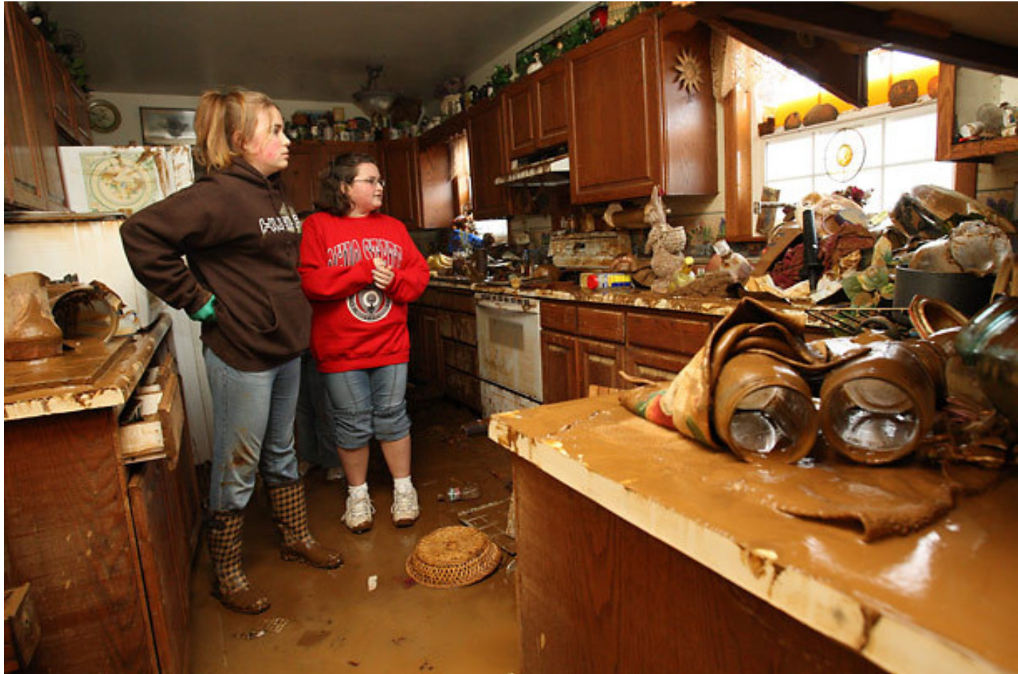
Curtis, WA, Aftermath of 7 Feet of Water STEVE RINGMAN / SEATTLE TIMES
