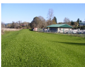
Pe Ell Wastewater Treatment Plant Flood Protection Dike
