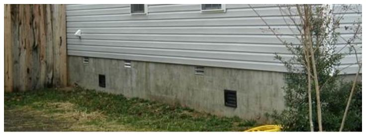
Example of Completed Retrofit (foundation has both air and flood vents)
