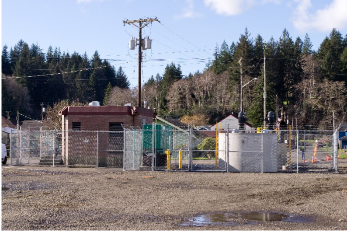
Ramer Street Pump Station (pic 1):
