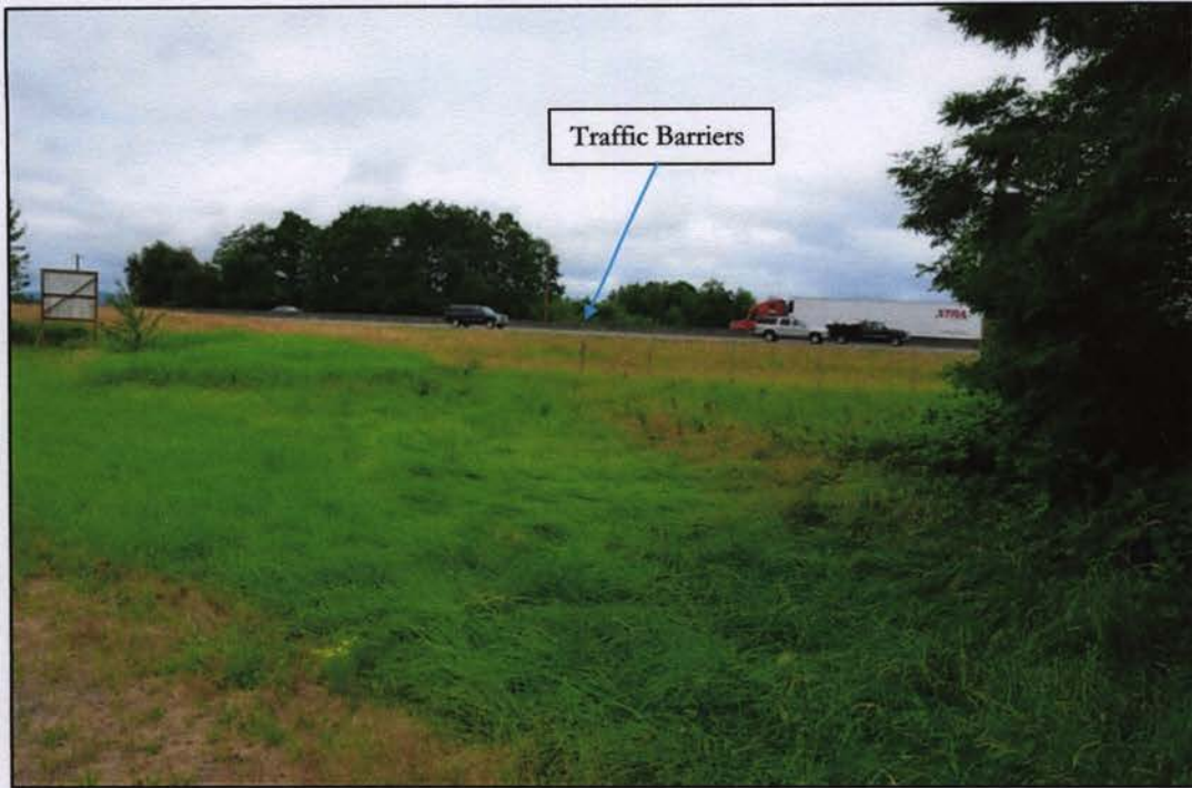
Figure 3. Center barriers along I-5.
