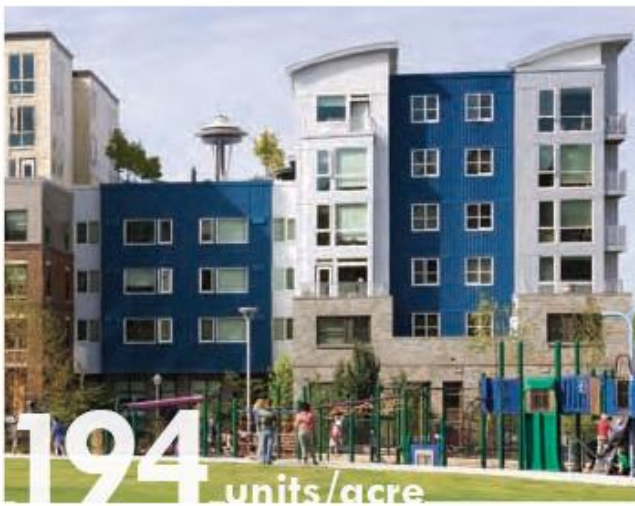
The Alcyone mixed-use development in Seattle's South Lake Union neighborhood provides 161 mixed-income apartments on 0.83 acres for a net density of 194 units per acre.
