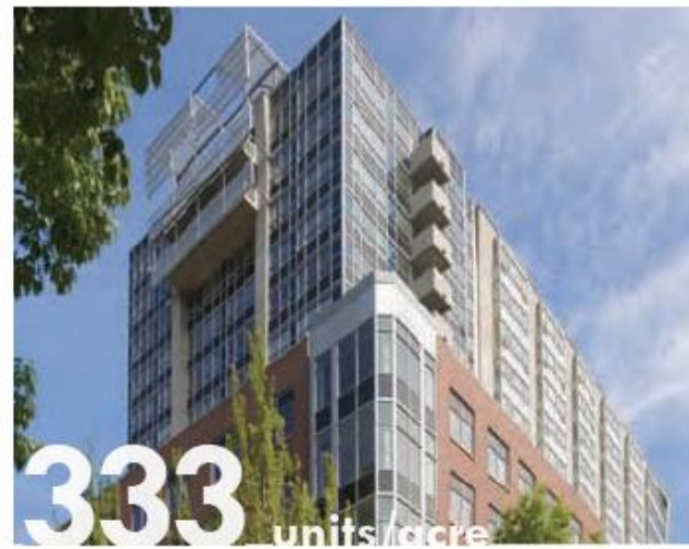
The 18-story M Street mixed-use development in Seattle's First Hill neighborhood provides 220 market-rate apartments on 0.66 acres for a net density of 333 units per acre.
