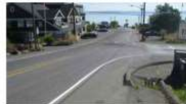
Existing Site - Main at Colchester Drive
