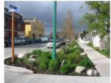
Bioretention facility, Water Street, Pt. Townsend, WA
