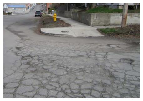
Alligator cracking: Alligator cracking is called such because it resembles the pattern on an alligator It is generally skin. located within the wheel path of the travel lanes and is caused by traffic loads. Alligator cracking is typically a sign of the base course and/or subgrade failing and starts as longitudinal cracks. Alligator cracking can be a serious problem and lead to rapid deterioration of the street.
