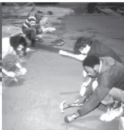
(Left) Templates installed every two and a half feet for the construction of the model, between which the concrete was poured and contoured. (Right) Model aides installing some of the 700,000 resistance strips.
