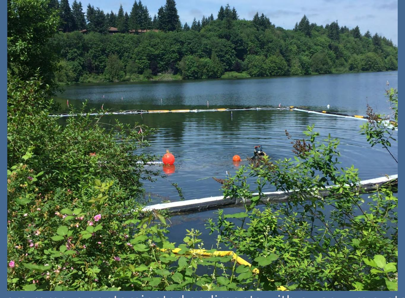
Divers remove contaminated sediments with a vacuum system
