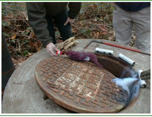
Different colored smoke candles used in a manhole (Photo Credit: Herrera).
