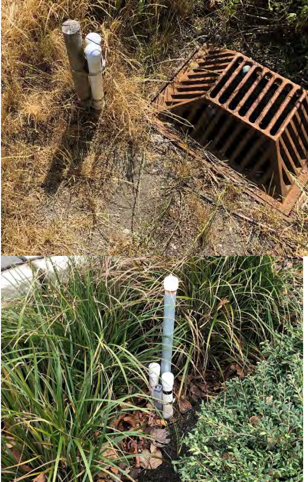
Figure 6. a) Ponding Wells at Overflow of TWH and b) Near Center of BCK
