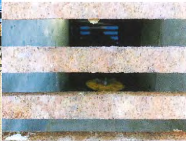
Plugged area drain to infiltration trench #1
