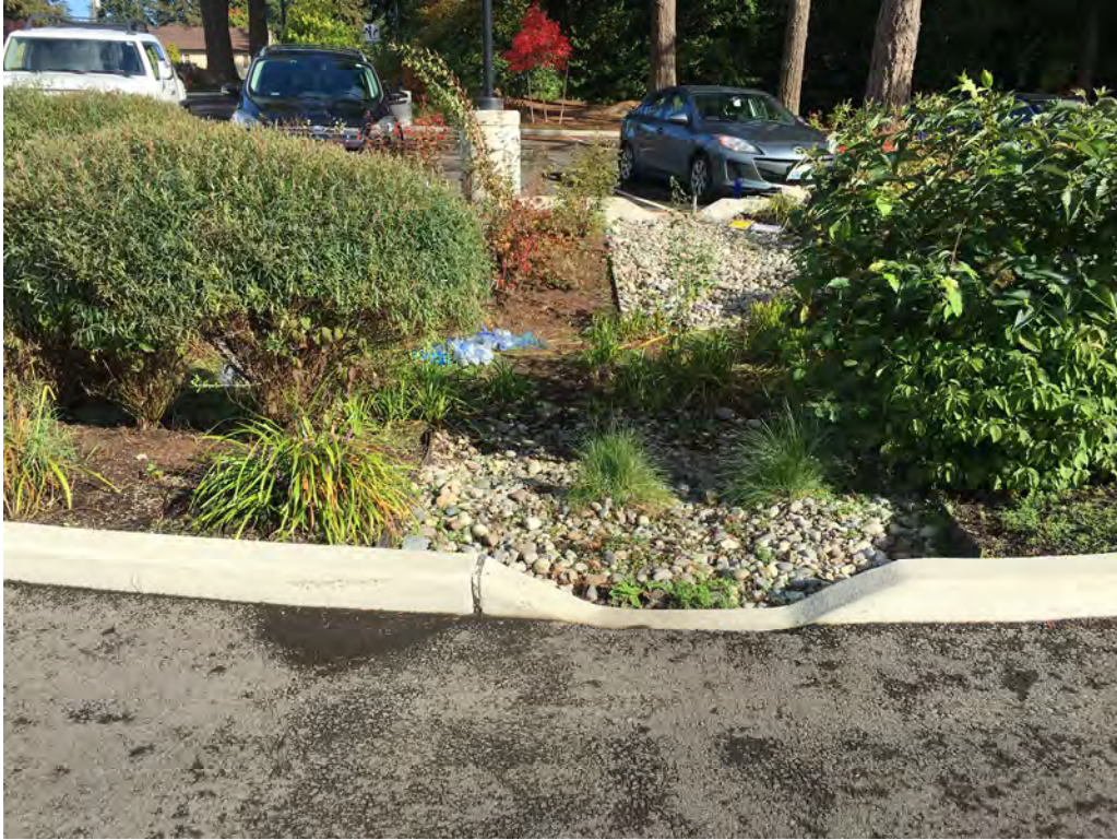
Cell FWI, curb cut inlet. Above photo is prior to install of weir. Lower photo is after weir install and during infiltration testing.
