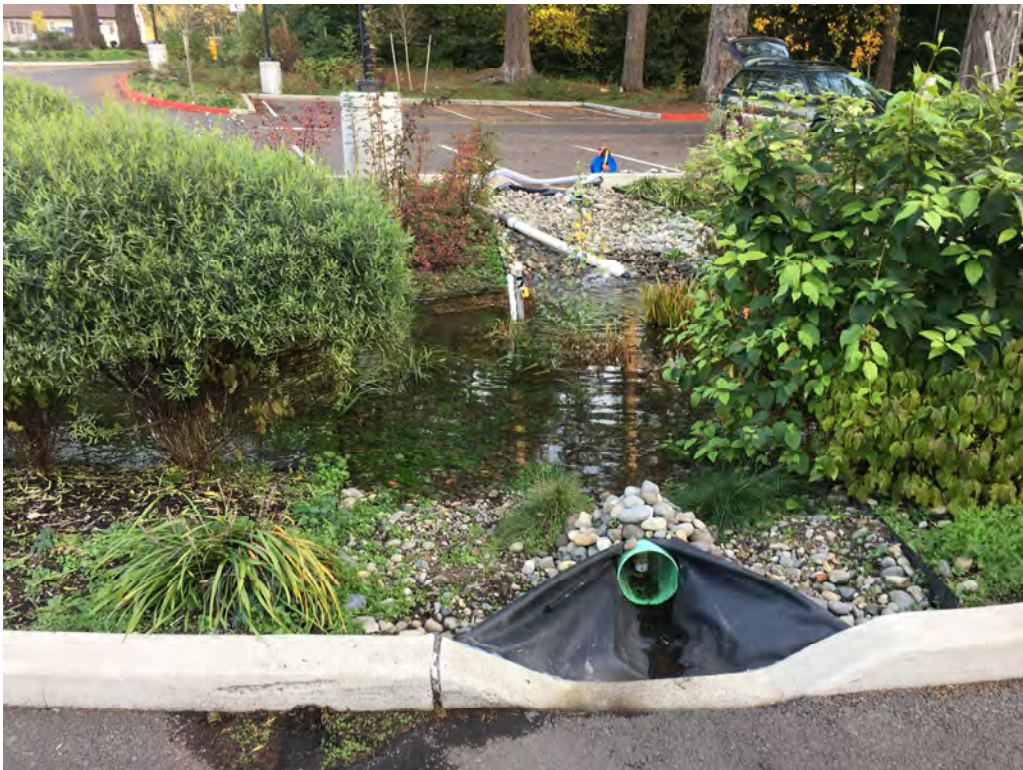
Cell FWI, curb cut inlet. Above photo is prior to install of weir. Lower photo is after weir install and during infiltration testing.
