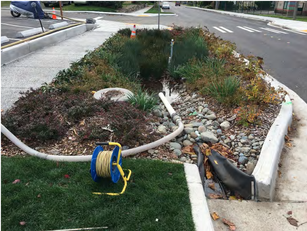
Cell RSH, primary curb cut inlet. Above photo is prior to install of weir. Lower photo is after weir install and during infiltration testing. Well point visible.
