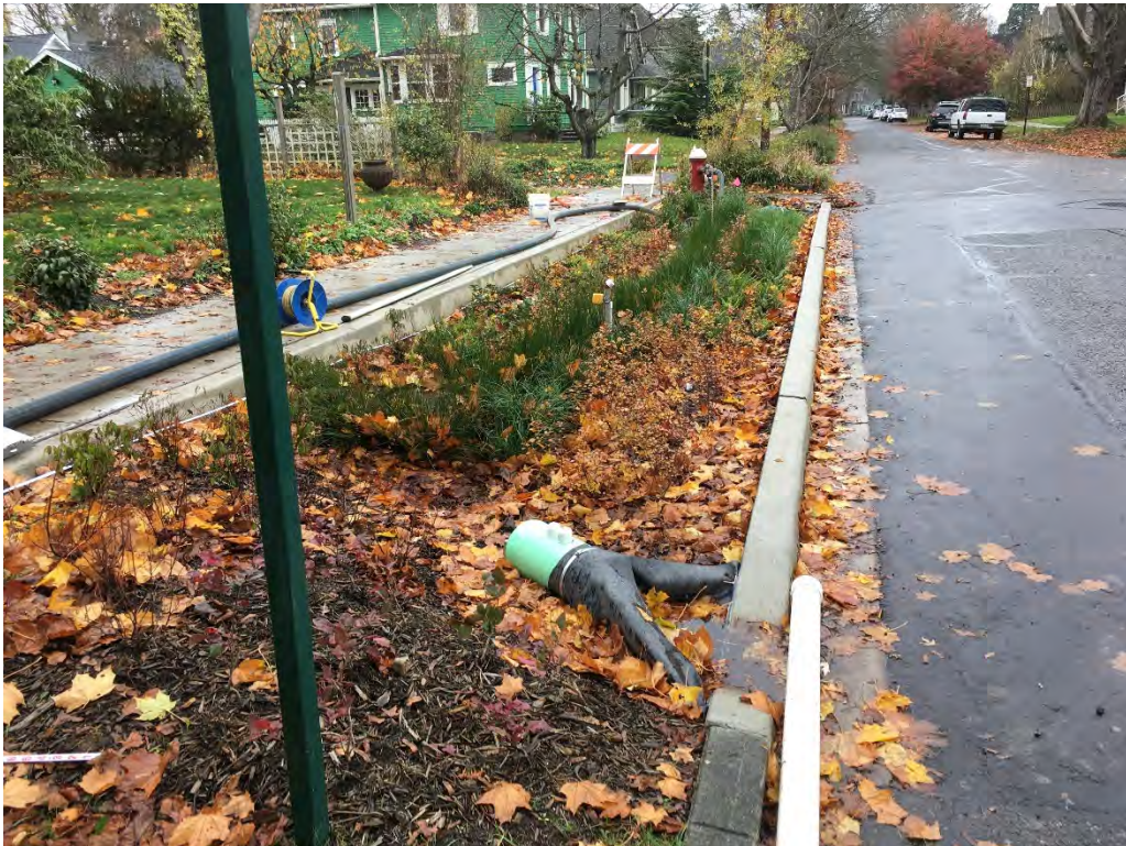
Cell BUW, primary curb cut inlet. Above photo is prior to install of weir. Lower photo is after weir install and during infiltration testing.
