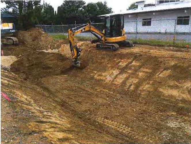
Photo 1 (left): Excavation of Bioretention Cell #6 in progress.
