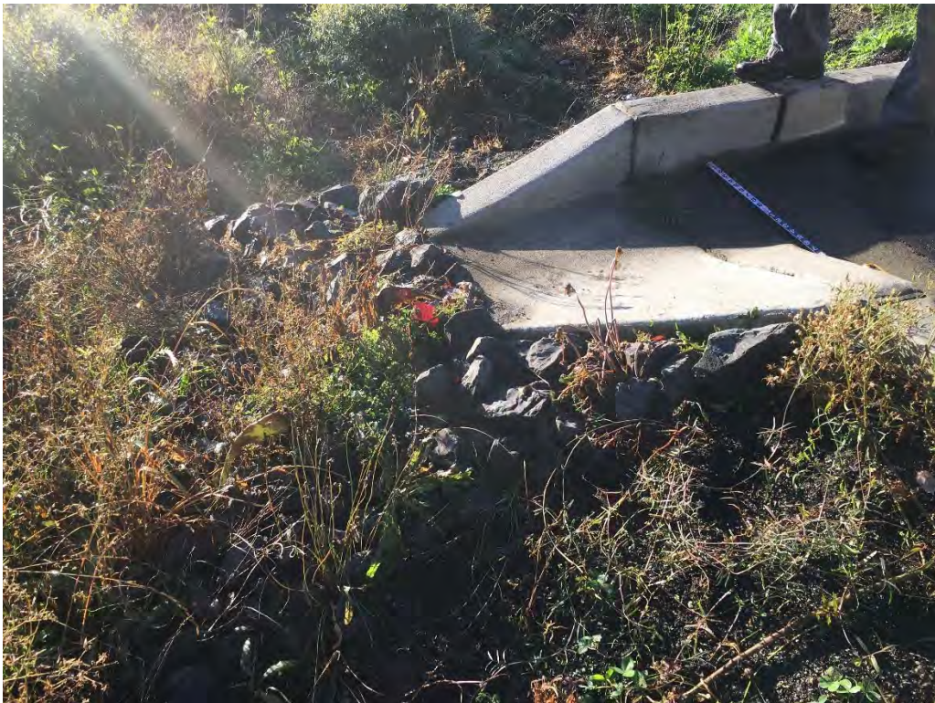
Cell TBM, curb cut inlet.
