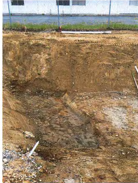
Photo 2 (right): Area excavated an additional ~0.5' at the north end of the cell.
