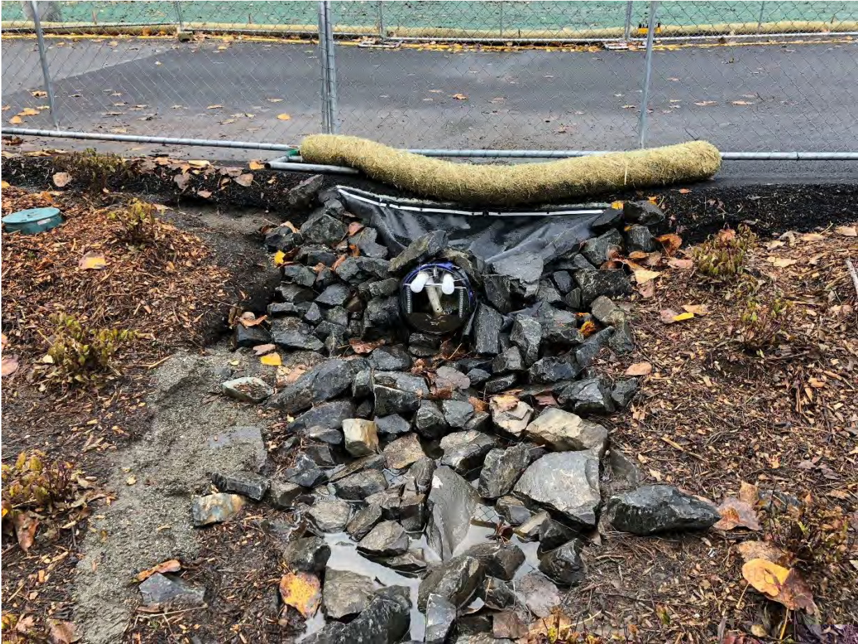
Figure 16. SSW_IN with Construction Wattle on November 6, 2018
