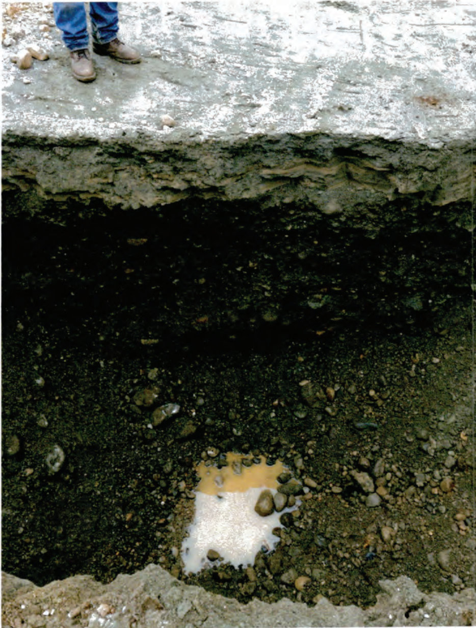
Picture 1: Bioretention Cell #3 excavation showing existing subgrade (310.5'), silt layer, underlying gravel, and groundwater.
