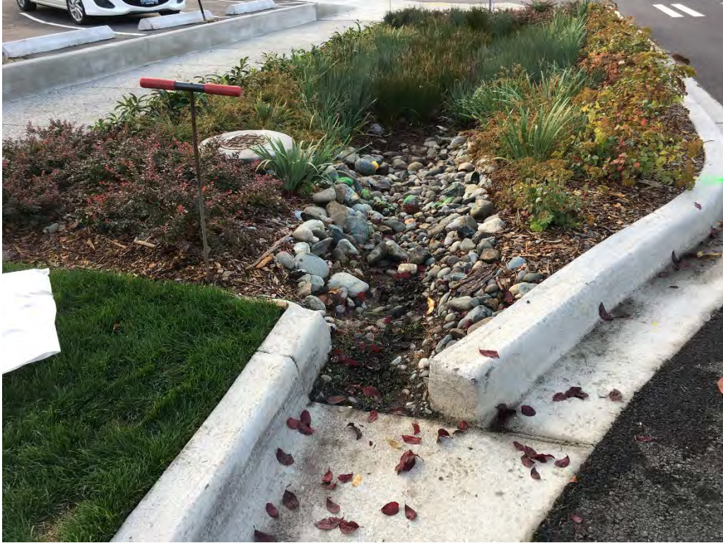
Cell RSH, primary curb cut inlet. Above photo is prior to install of weir. Lower photo is after weir install and during infiltration testing. Well point visible.
