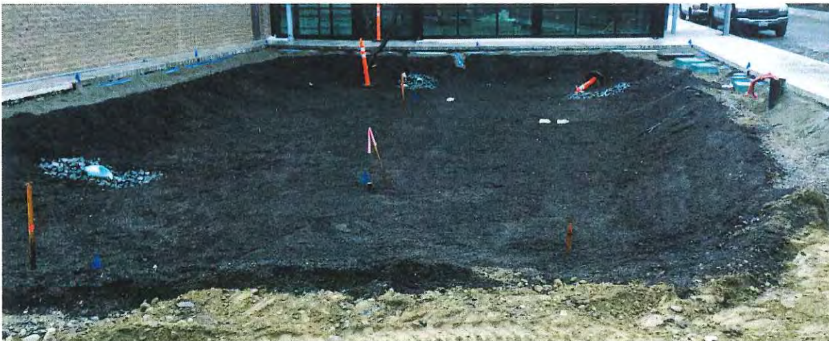
BR5, viewing north.
