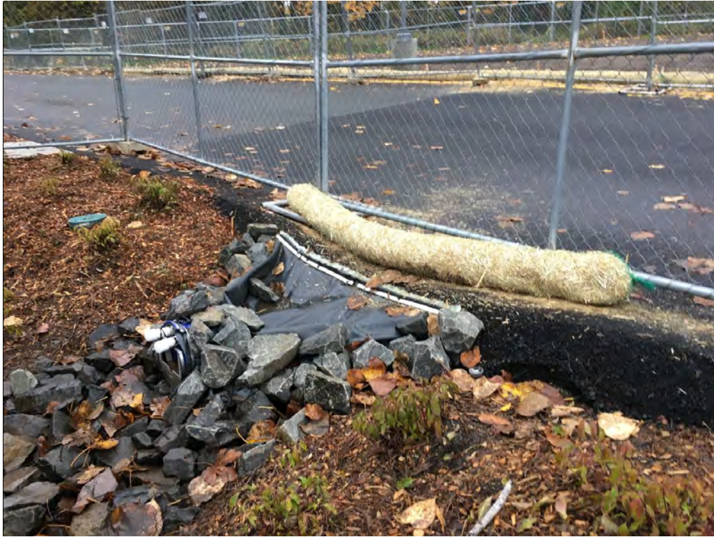
Above photo: Cell SSW inlet modified for monitoring. Note straw waddle attempt to limit turbid inflow. Lower Photo: close up of curb cut inlet prior to weir installation. Well point in foreground.
