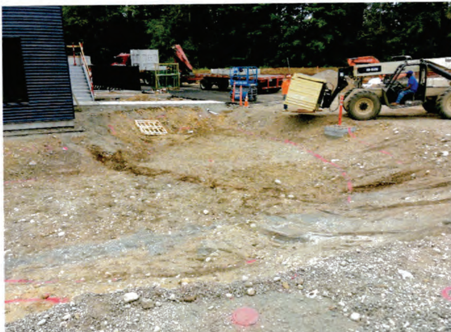
Picture 5: [Looking S/SW] BC-2 bottom of cell.
