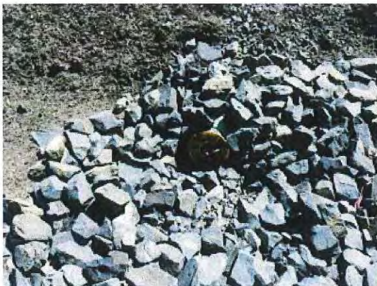
Area drain plugged to cell # 10
