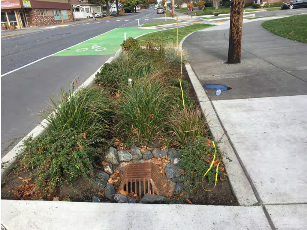
Cell BCK overview, overflow in lower center of photo
