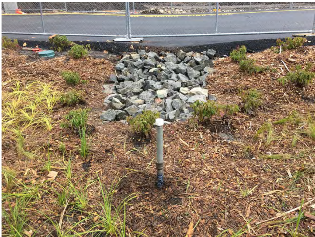
Above photo: Cell SSW inlet modified for monitoring. Note straw waddle attempt to limit turbid inflow. Lower Photo: close up of curb cut inlet prior to weir installation. Well point in foreground.
