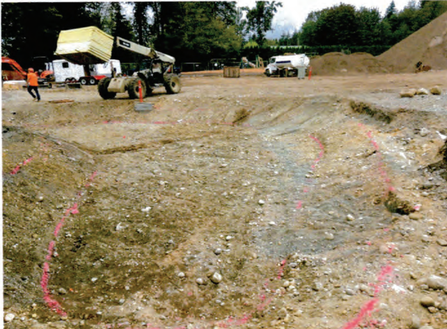
Picture 4: [Looking W] BC-2 bottom of cell
