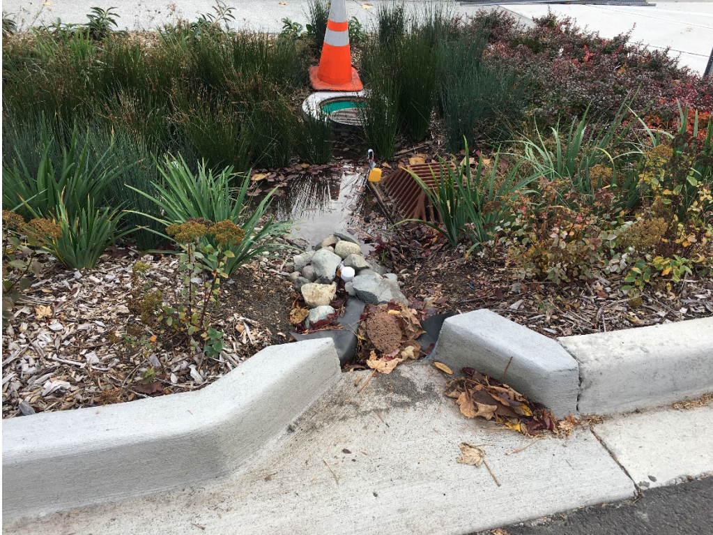
Above photo: RSH secondary curbcut. Overflow beehive visible in vegetation. Orange cone next to drain basin structure. Lower Photo: view of secondary curbcut, overflow and drain basin.
