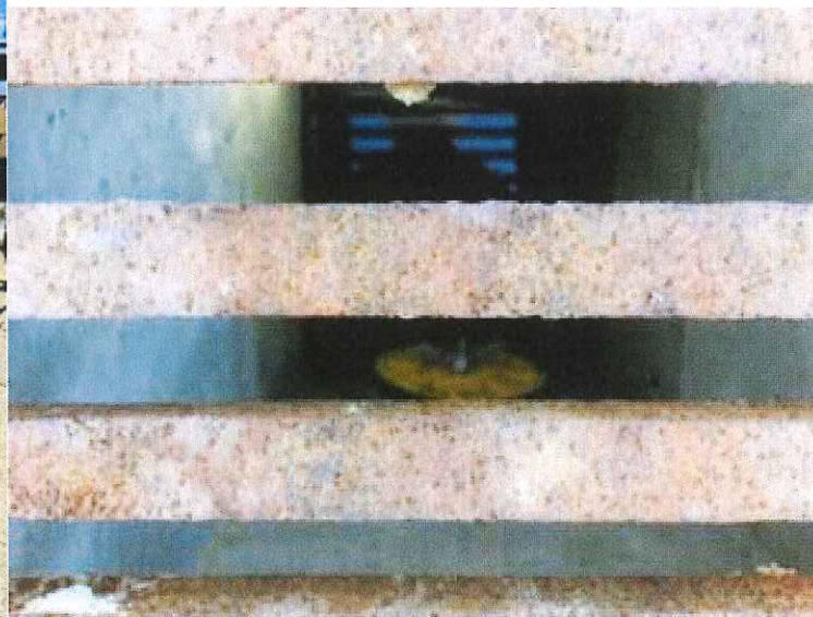
Plugged area drain to infiltration trench #1
