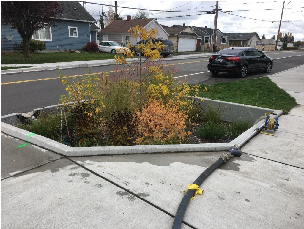
Cell M3Q overview. In above photo, the curbcut weir has not been installed. Lower photo is after weir install and during infiltration testing.
