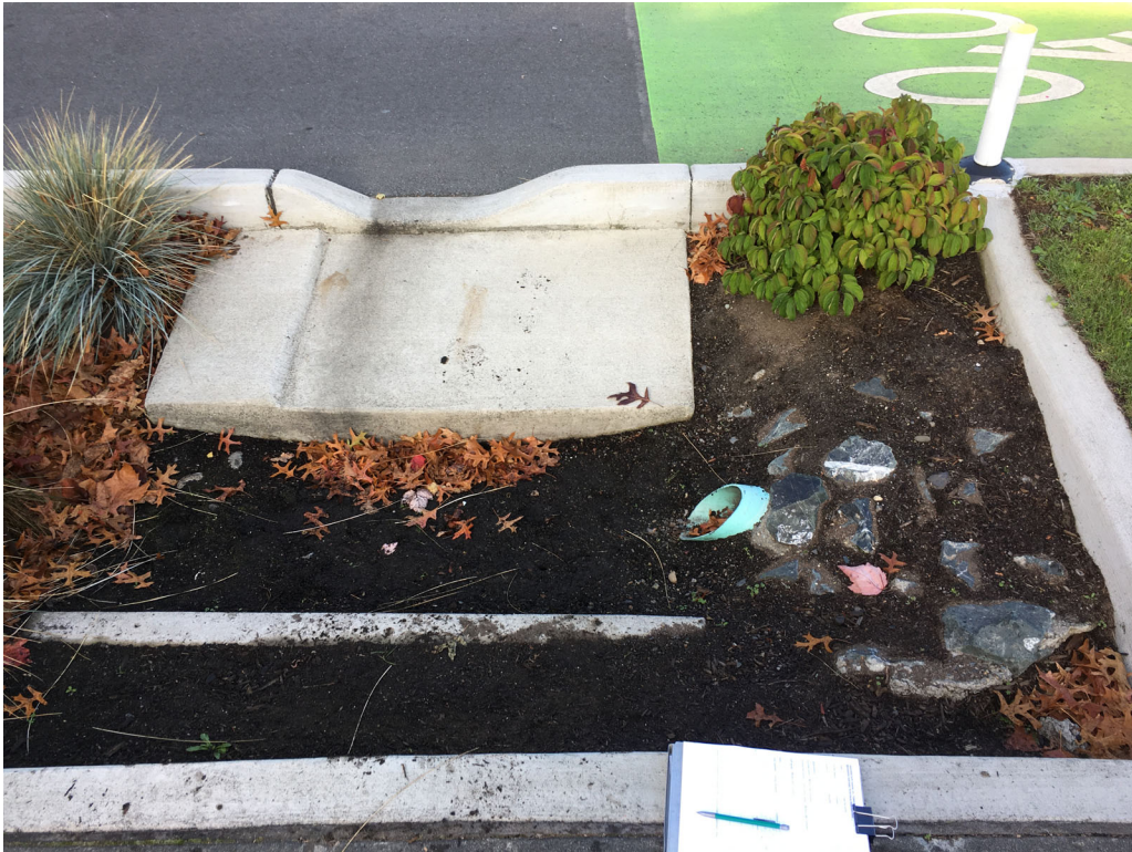
Cell BCK, curb cut inlet and undocumented inlet (green pipe). Above photo is prior to install of weir. Lower photo is after weir install and during infiltration testing.
