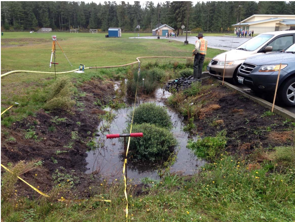
Cell TBM during infiltration testing, looking southeast, after about 1.5 hours of inflow.
