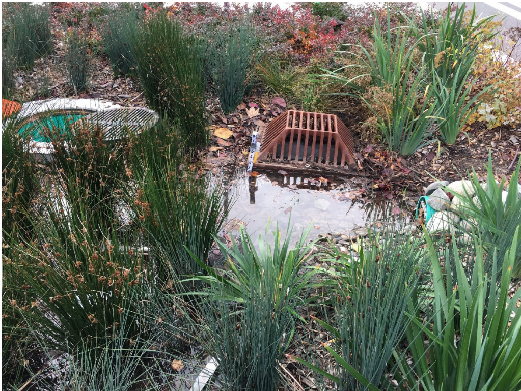
Above photo: RSH secondary curbcut. Overflow beehive visible in vegetation. Orange cone next to drain basin structure. Lower Photo: view of secondary curbcut, overflow and drain basin.
