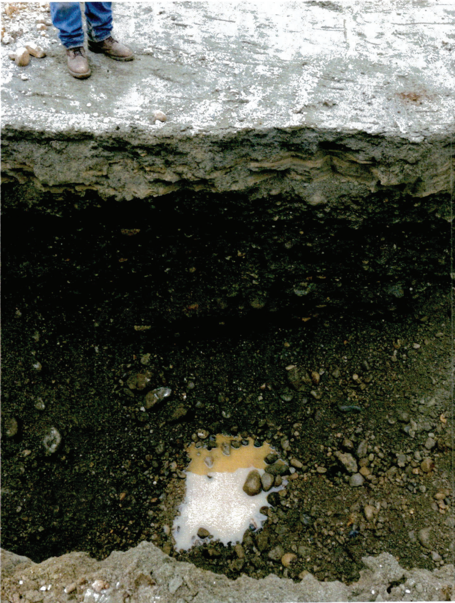
Picture 1: Bioretention Cell #3 excavation showing existing subgrade (310.5'), silt layer, underlying gravel, and groundwater.
