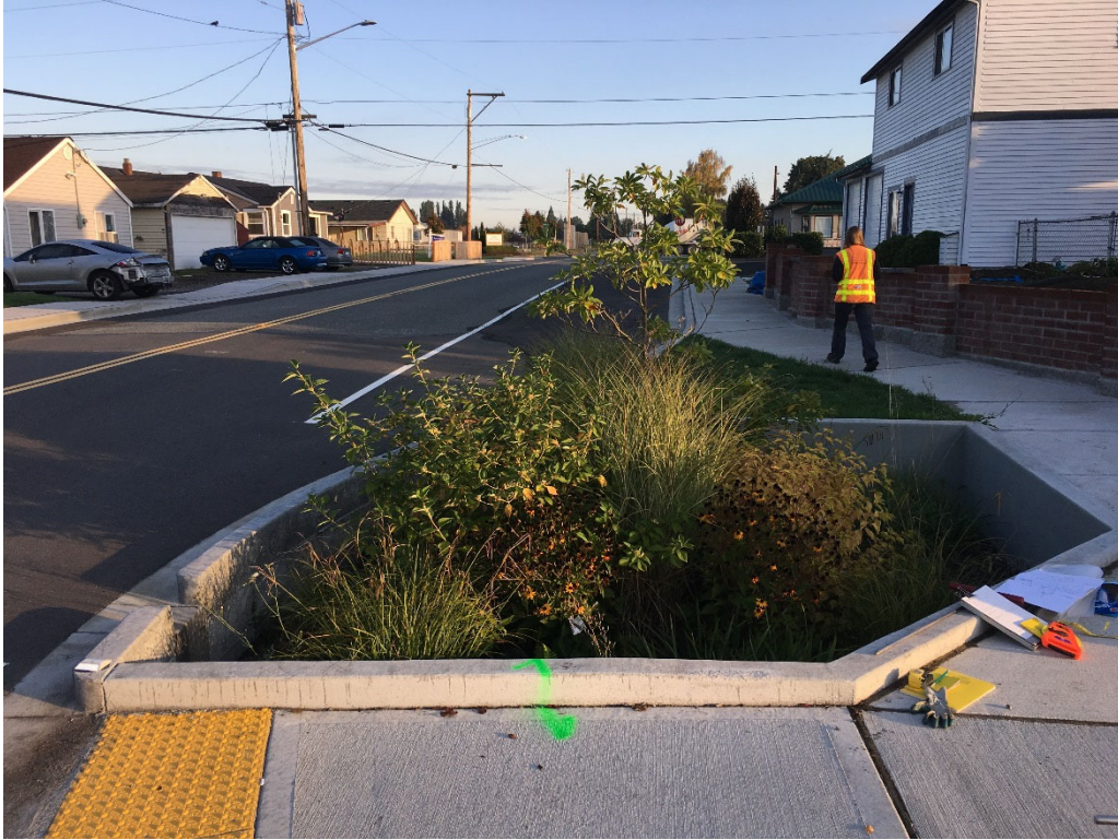
Cell M3Q overview. In above photo, the curbcut weir has not been installed. Lower photo is after weir install and during infiltration testing.
