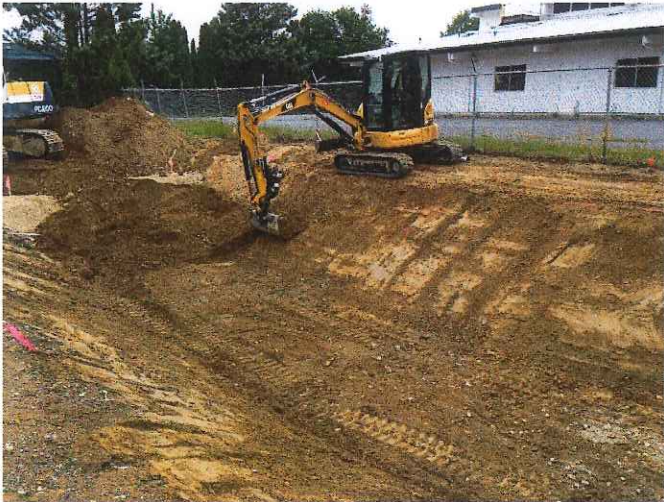
Photo 1 (left): Excavation of Bioretention Cell #6 in progress.
