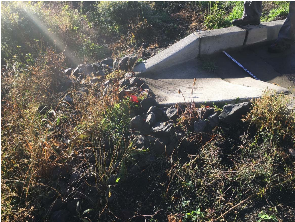
Cell TBM, curb cut inlet.
