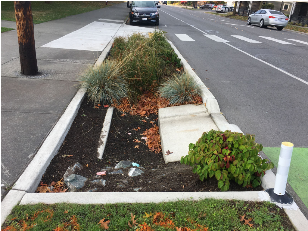
Cell BCK overview, curbcut inlet shown
