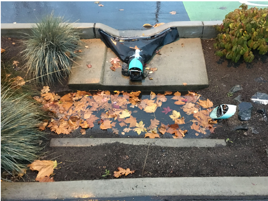
Cell BCK, curb cut inlet and undocumented inlet (green pipe). Above photo is prior to install of weir. Lower photo is after weir install and during infiltration testing.
