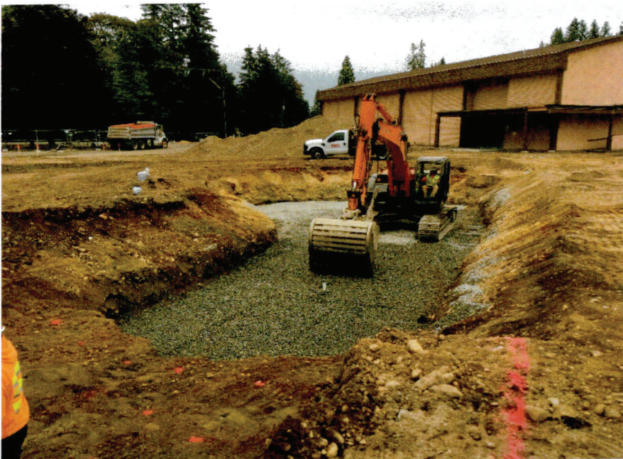
Picture 3: [Looking S] BC-3 Top of drain rock.
