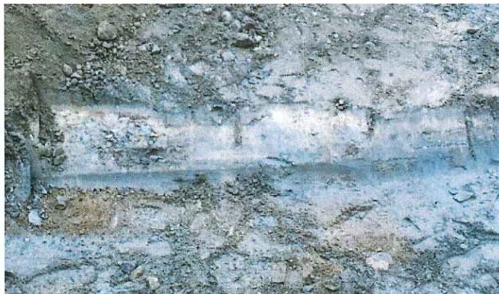
Left: Looking south at bioretention cell #6 subgrade. Right: Close-up of ridge of in-place silty material.
