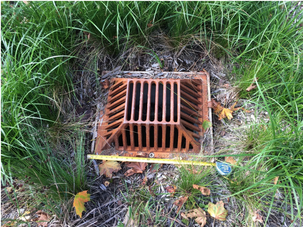
Above photo: BUW secondary curbcut. Overflow beehive just visible in vegetation, upper right. Lower Photo: close up of overflow structure.
