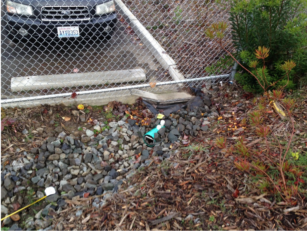
Above photo: Cell MPP inlet modified for monitoring. Lower Photo: close up of curb cut inlet prior to weir installation.
