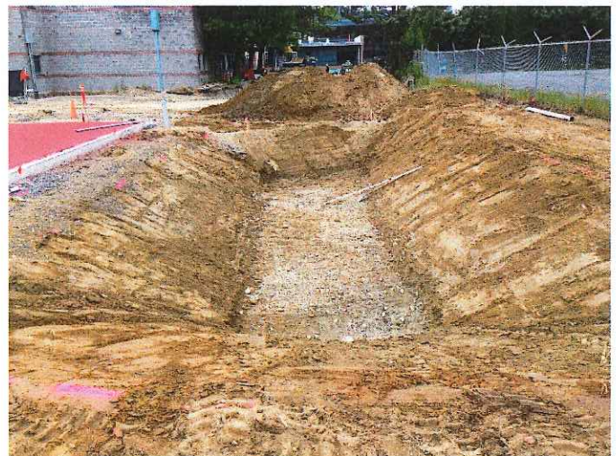
Photo 4 (right): Bioretention Cell #6 viewed from the south.
