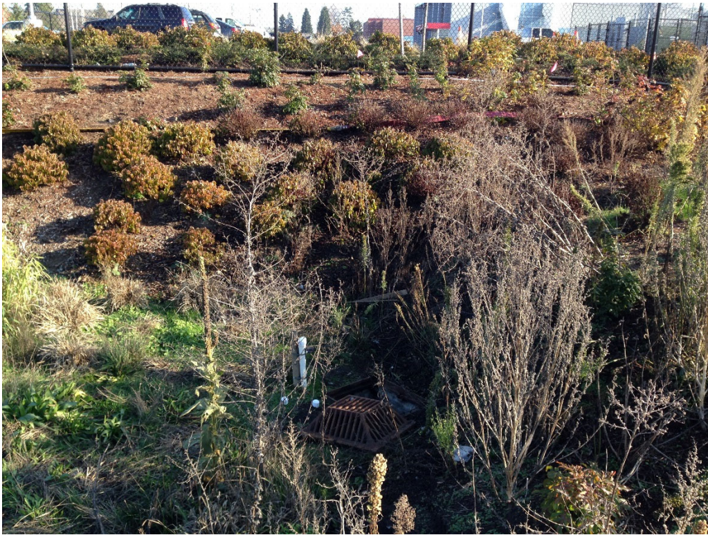
Lower Photo: overflow structure.
