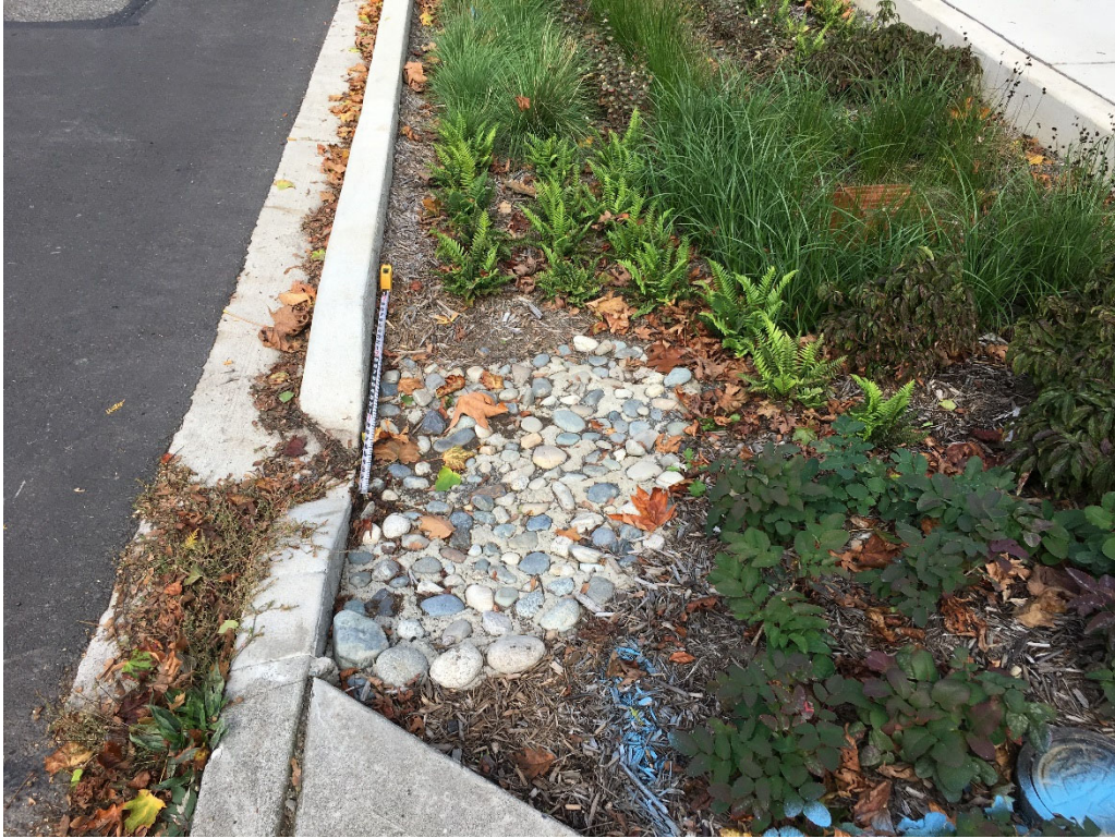
Above photo: BUW secondary curbcut. Overflow beehive just visible in vegetation, upper right. Lower Photo: close up of overflow structure.
