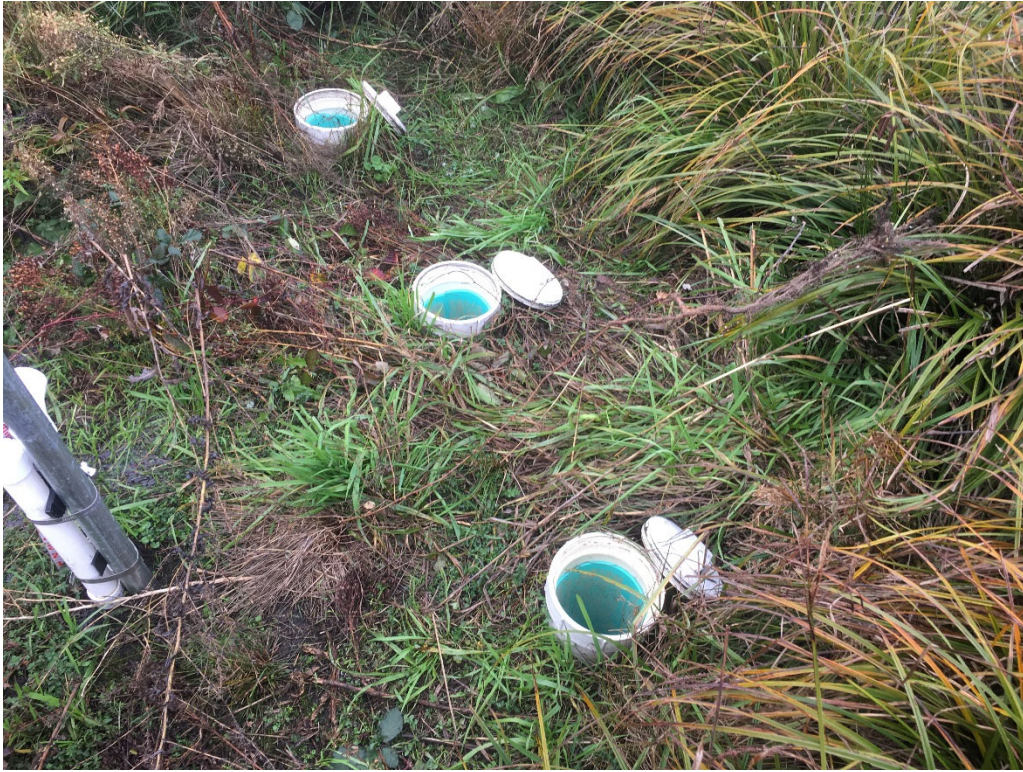
Above photo: TWH, underdrain cleanouts and well point.
