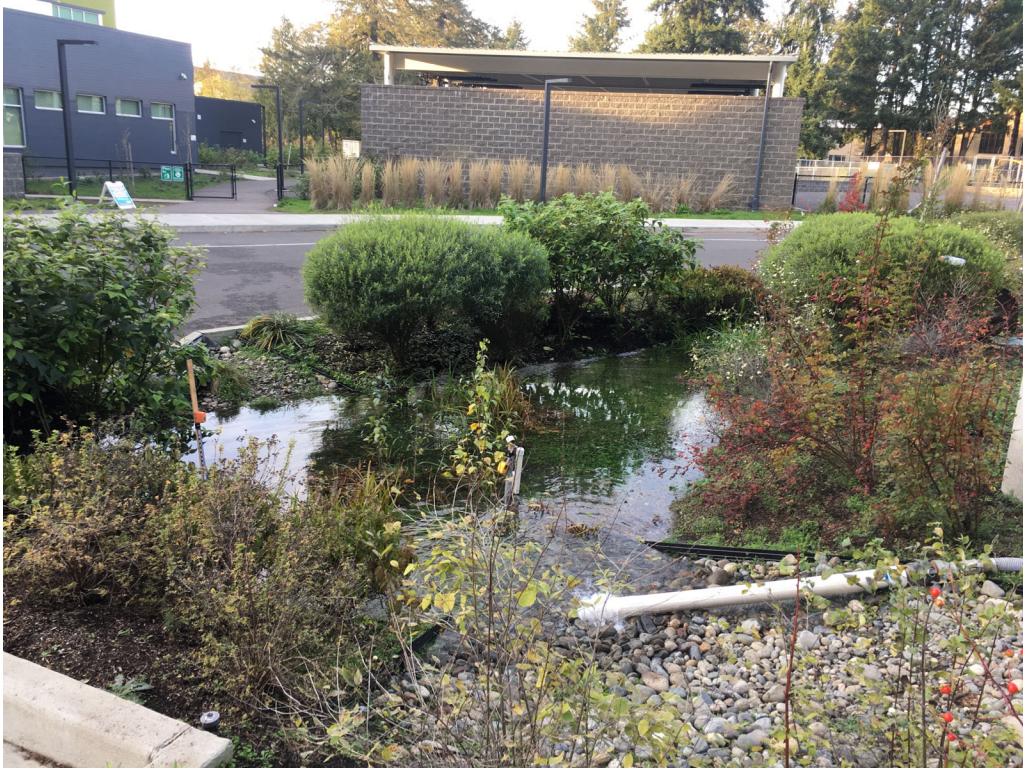
Above photo: FWI during infiltration testing. Overflow beehive not visible in vegetation, located in lower left. Lower Photo: overflow structure and staff gauges.
