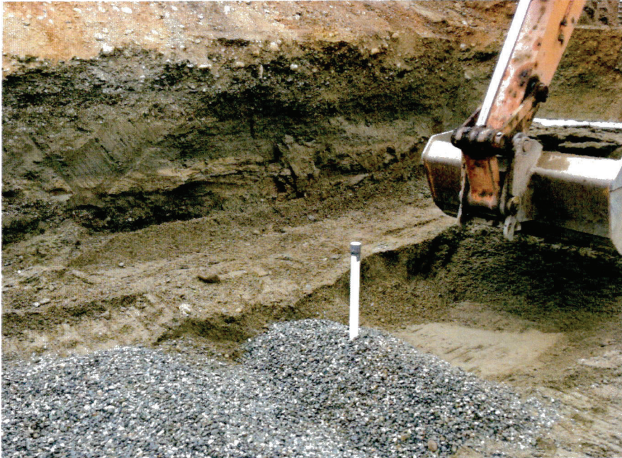
Picture 2: [Looking NW] BC-3 installation of 2" PVC for piezometer in pit drain area. Subgrade at northern end of infiltration region is a sand rather than a gravel.
