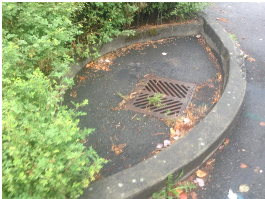
Overflow structure in Cell BDP
