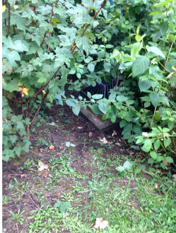
Cell NOL overflow structure
