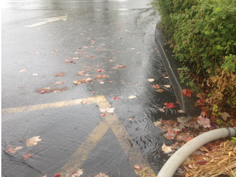
Diversion of stormwater flow to street during storm event during infiltration testing, due to leaf litter collected in curb cut
