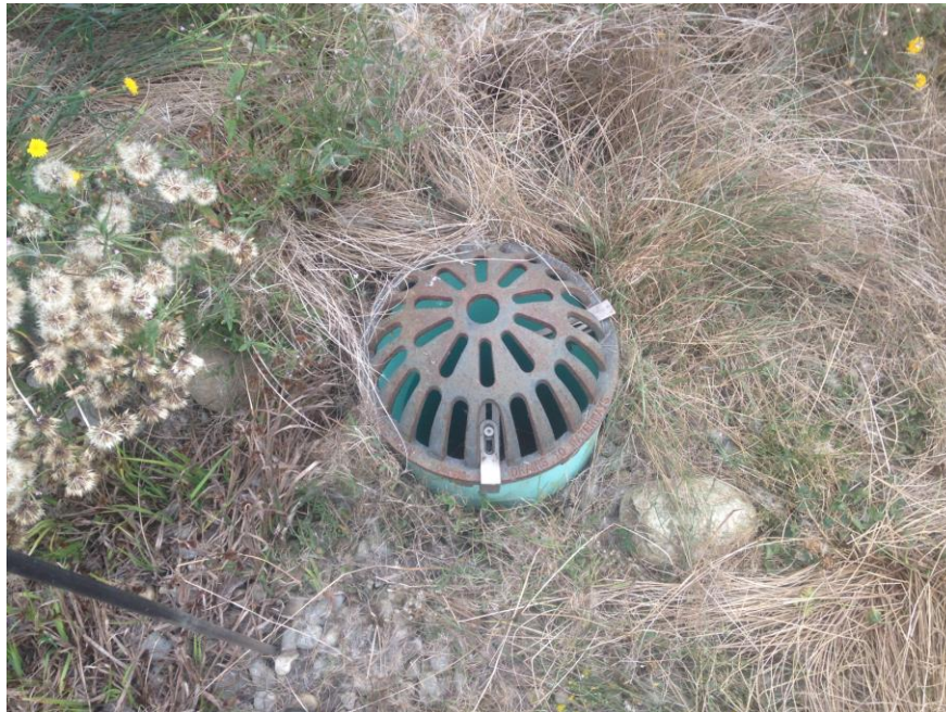
Overflow structure in Cell ORLA1-B
