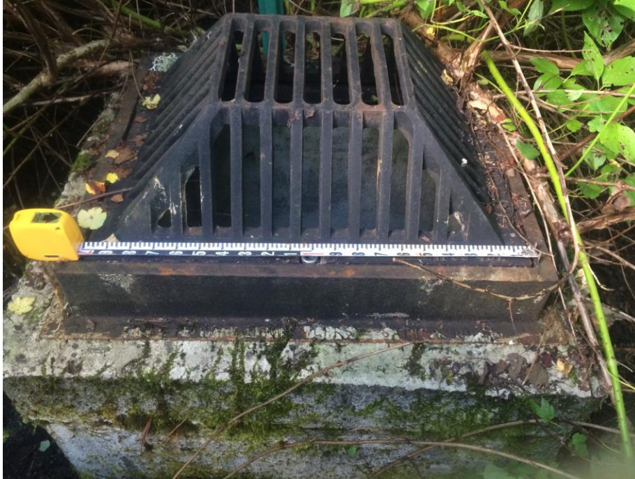
Cell IHS overflow structure
