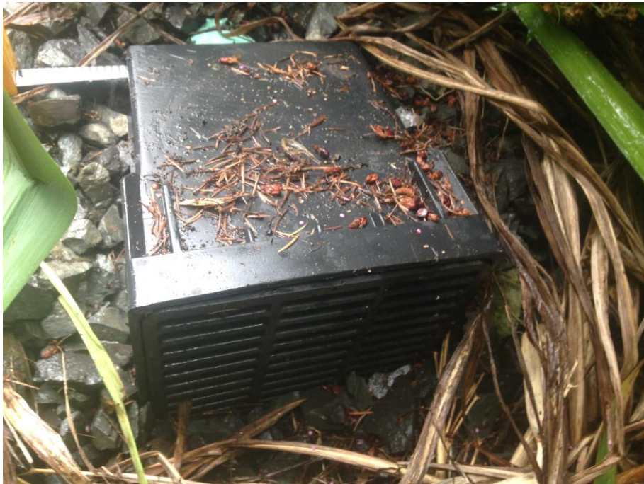
Overflow structure in Cell MCCA1
