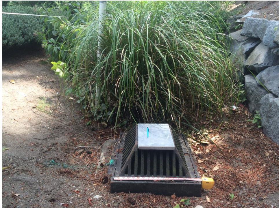
Cell B145 overflow structure and pre-existing piezometer
