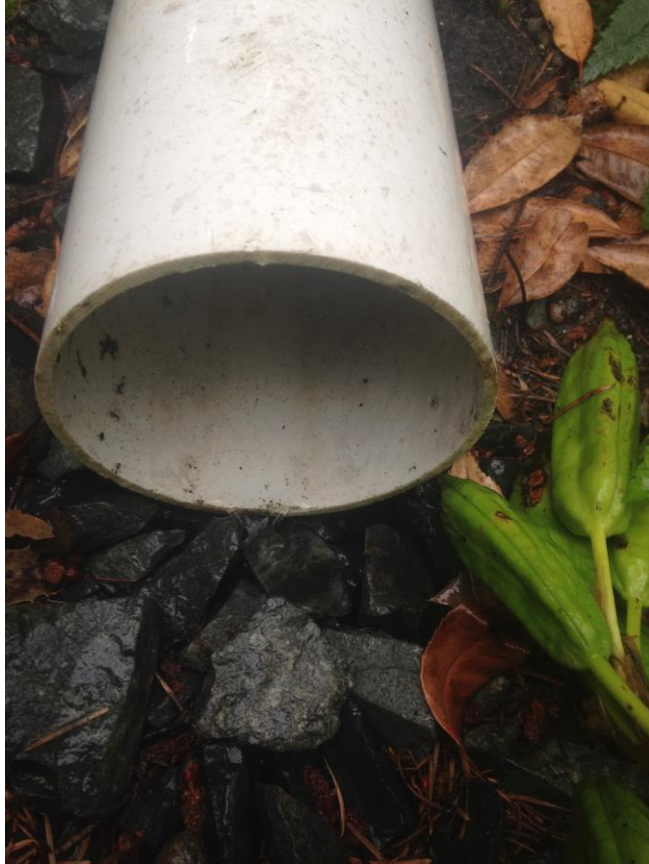
Flow from inlet to MCCA2 during beginning of infiltration testing, with some flow visible
