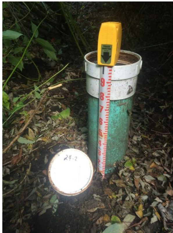
Cell IHS pre-existing piezometer 24-2
