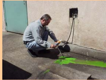
Bright-colored dyes are used to track stormwater flows
