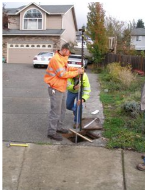
Catch basin inspection for depth of sediment accumulation.
