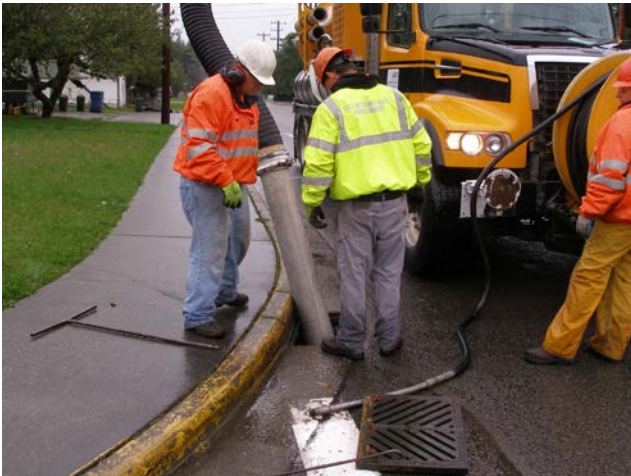
Vector truck crew cleaning out a catch basin.
