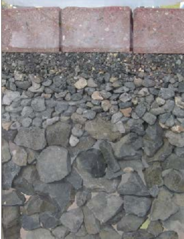
Figure 5. Cross section of permeable concrete pavers and underlying base course
