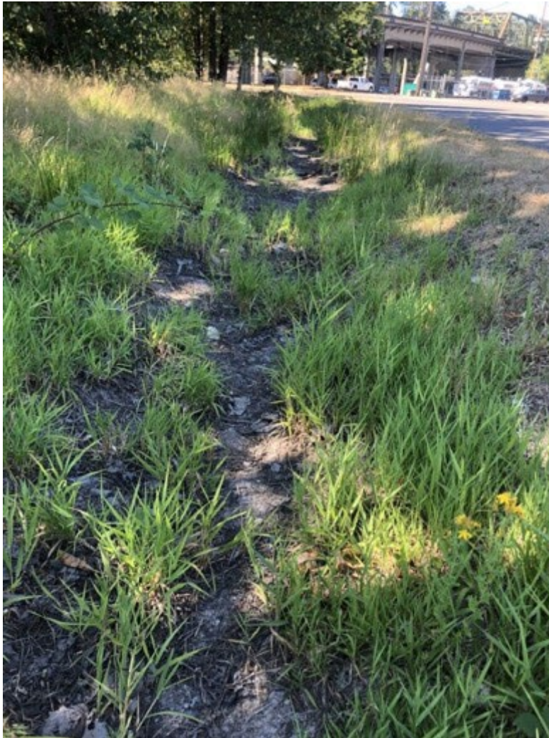
Figure 1. Fife ditch before renovation activities in 2019
