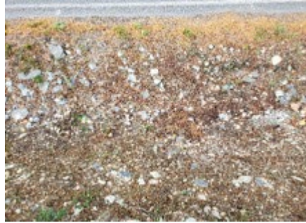
Figure 57. WSDOT Blend 78th Ave site 10/31/23
