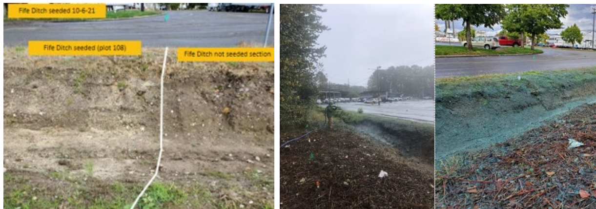
Figure 4. Seed applied to bare soil in each plot followed by the application of hydro mulch to stabilize the plot
