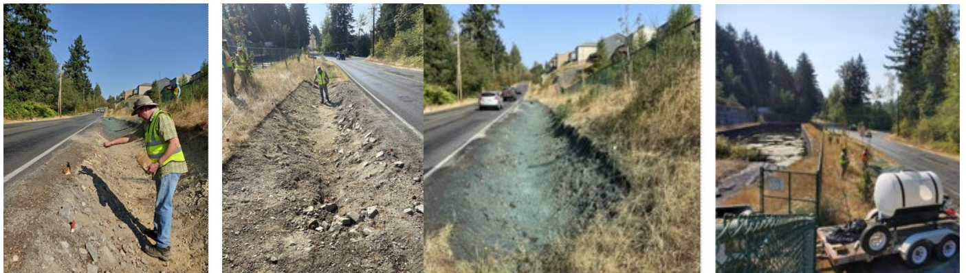
Figure 6. 78th Ave site seeding and hydro mulch. Seeding date 9/27/22
