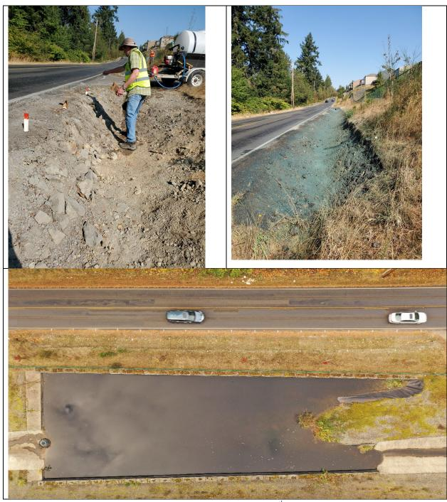
Figure 3: Construction and hydroseeding of plants in the 78<sup>th</sup> Ave Ditch. Lower row of images shows drone shoots of the site showing plan establishment.
