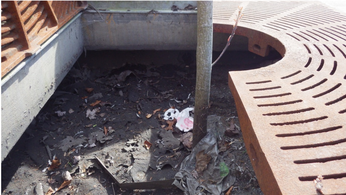
Figure J-3. Sediment at the top of Filterra media (April 4, 2014).
