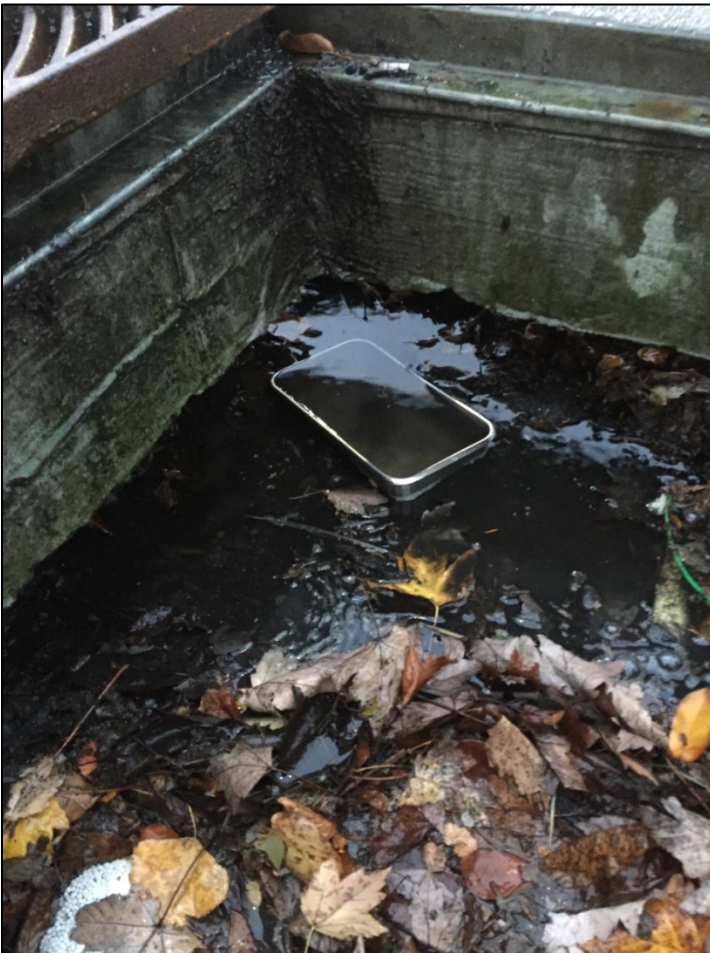
Figure C-2. Filterra inlet sampling, stainless steel tray collecting water from curb cut (October 26, 2016).
