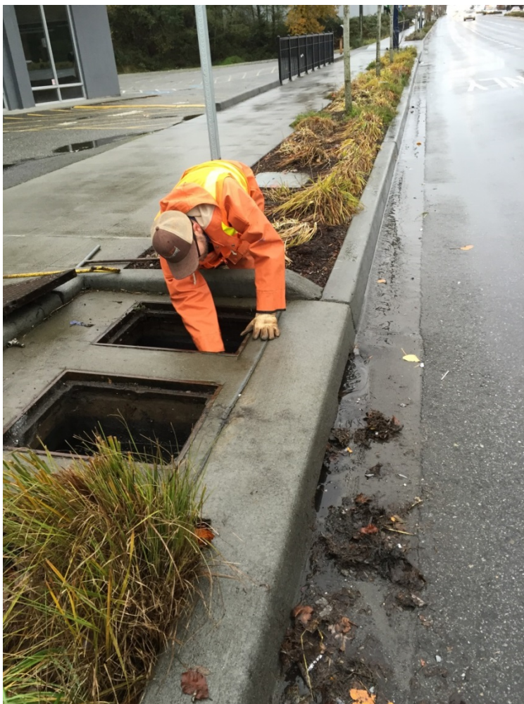
Figure J-2. Clearing debris blocking curb cuts at BPB1 inlet (December 3, 2015).
