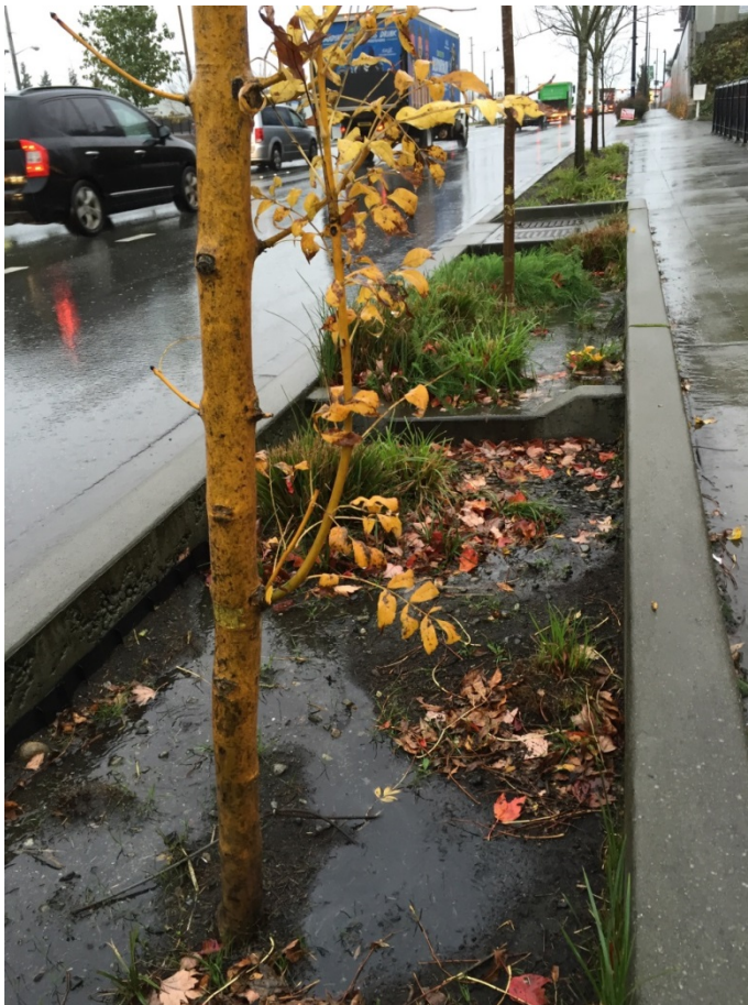
Figure J-3. Sparse vegetation and yellowed trees at BPB2 - this did not appear to affect performance (October 26, 2016).
