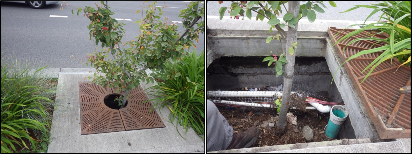
Figure C-1. Filterra with closed grate and Filterra with open grate, clean-out uncapped (June 2, 2015).
