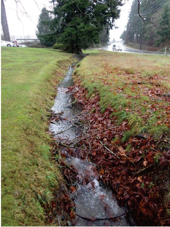
Figure 12. Ditch along South 356 th Street that carried stormwater runoff to bioretention facilities during the study period. In summer 2017 the ditch was replaced by pipes and a sidewalk after the study.
