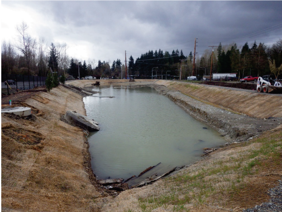
Figure 3. The new CDSTW under construction, March 31, 2014.
