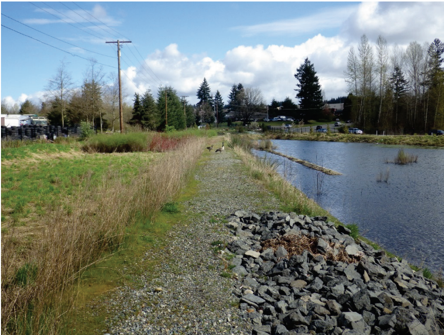
Figure 6. Established vegetation in west bioretention facility (on left) and new CDSTW (on right), March 24, 2016.
