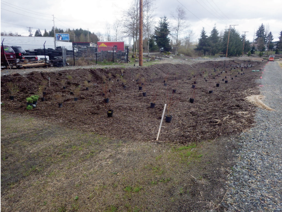
Figure 5. The west bioretention facility pre-planting, March 31, 2014.
