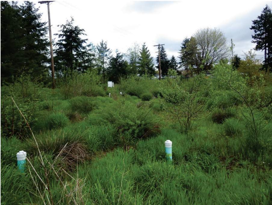
Figure 8. Mature vegetation in east bioretention facility, April 27, 2017.
