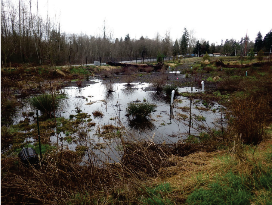
Figure 7. Immature vegetation in east bioretention facility prior to initiation of stormwater sampling, February 16, 2016.
