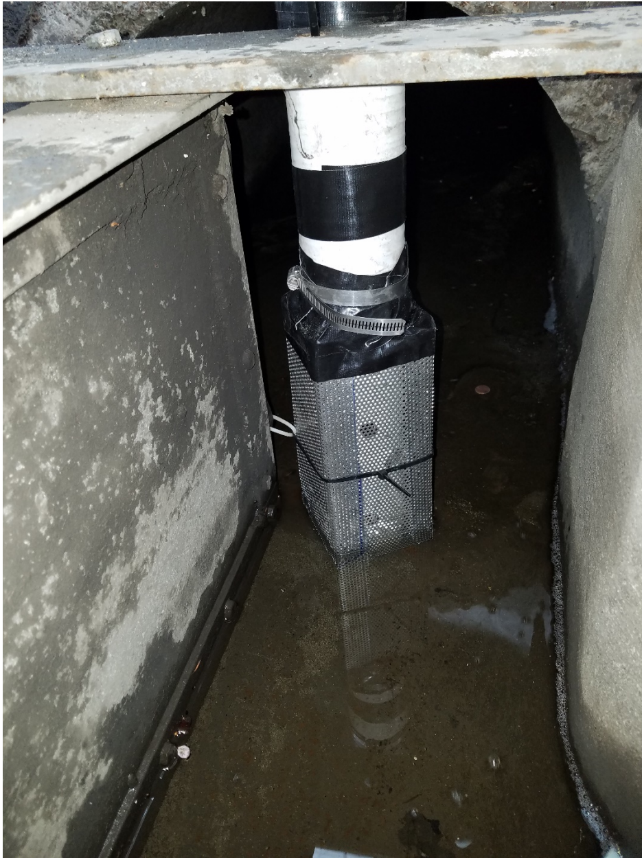
Figure 5-A. Inlet standpipe installed in the stormwater vault.
