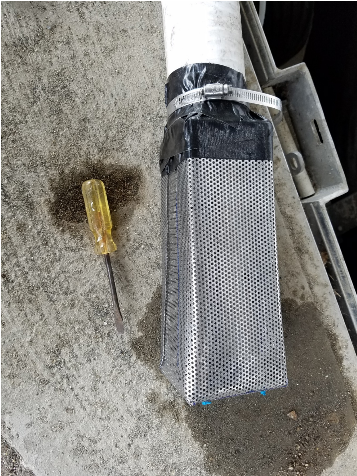
Figure 4-A. Completed standpipe for dosing pump inlet.
