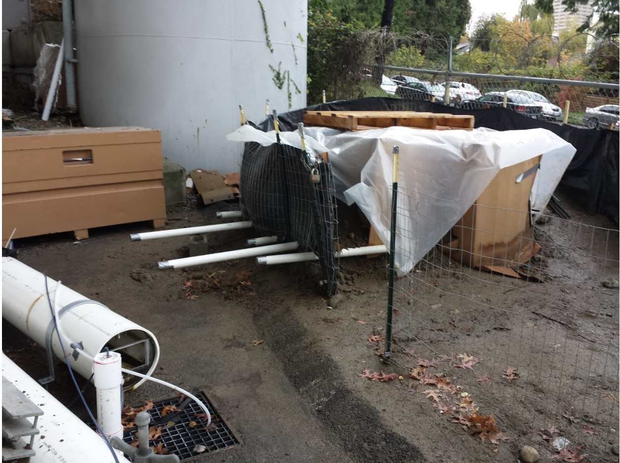
Figure 8-A. Mesocosms being buried in native soils to buffer temperature fluctuations. Effluent drains not trimmed to length or connected to the drain manifold.
