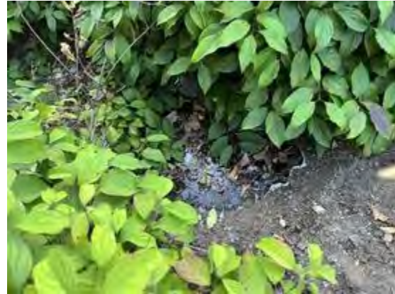
Site Photo: OutfallPonding.JPG
