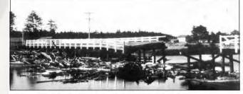
Figure 3. Photo 9-1-A. Two spans lost and timber bent. Two other 20-foot spans are shown considerably deflected. Map location 5.
