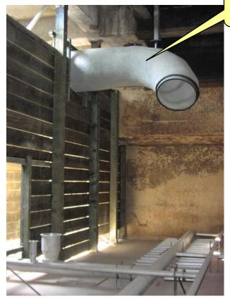
Piping and Baffles for Step Feed
