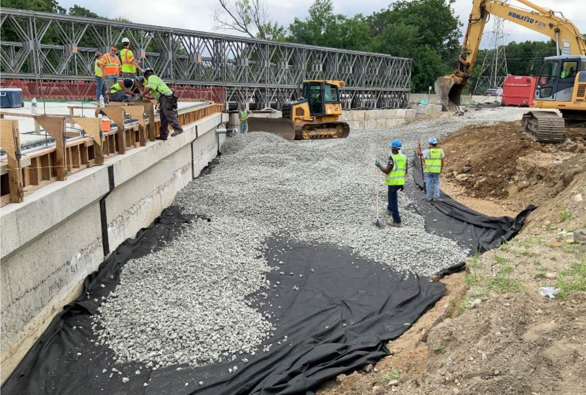
I-80 Bridges over Rockaway River, Denville, NJ
