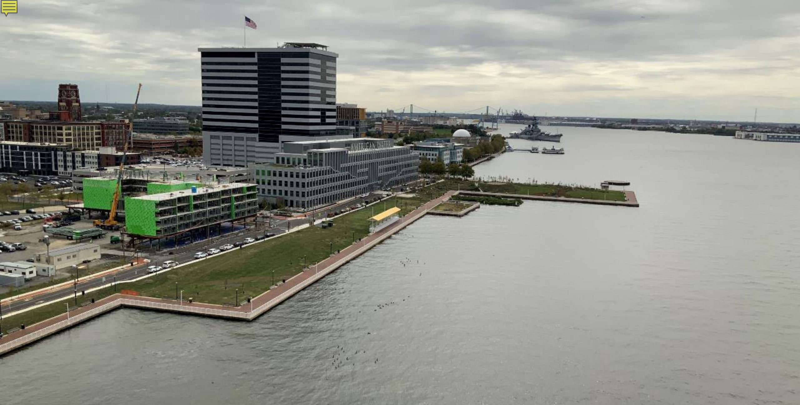
RCA Pier and Hilton Garden Inn, Camden, NJ
