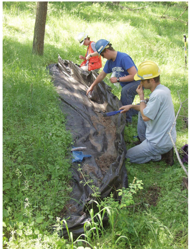
Figure 2. Example of a sediment fence. The fence is 5 meters wide, 0.5 m tall, with a 0.8 m long apron. The upslope edge of the apron is buried in a shallow trench. See Robichaud and Brown (2002) for installation details.
