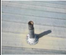
Photograph 9: Lead flashing around classroom building roof penetration.
