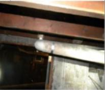
Photograph 12: ACM hard mud pipe fitting insulation on fiberglass insulated pipes in crawlspace.
