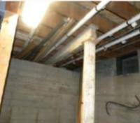
Photograph 6: ACM Aerocel pipe insulation in lunchroom basement.
