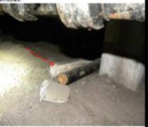
Photograph 10: ACM hot water pipe insulation debris on crawlspace floor.
