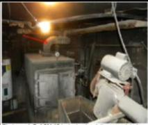
Photograph 7: ACM 10 inch pipe insulation associated with boiler.
