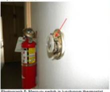
Photograph 5: Mercury switch in lunchroom thermostat.
