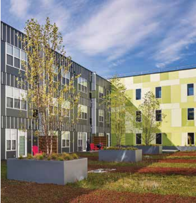
Paseo Verde, a 120-unit mixed-income development in North Philadelphia, has a green roof over the first level that minimizes runoff and doubles as garden courtyards, an attractive amenity for residents. (Halkin Mason Photography)
