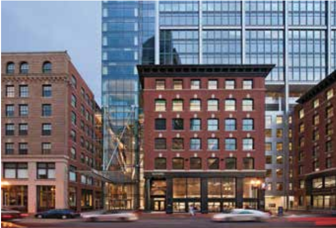
Atlantic Wharf, Boston's first green skyscraper, renovated and integrated 42 percent of the existing historic structures, including streetscapes and facades. (Anton Grassl/Esto)
