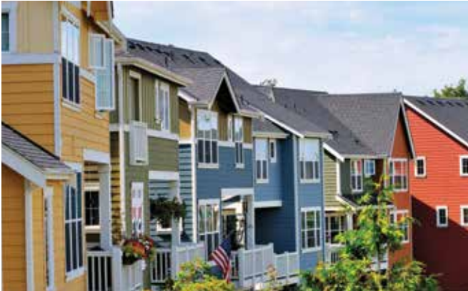
Located on the site of a former public housing complex once marked by crime and unemployment, High Point includes more than 1,500 homes, of which 48 percent are affordable for low-income families. (© Juan Hernandez for Mithun)
