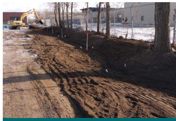
Figure 2.8.4: During the Bernardi retrofit the buffer strips were excavated and compacted topsoils were disposed. (Source: Aquafor Beech)
