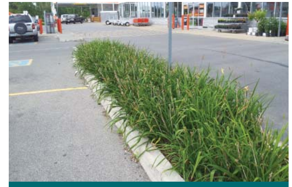
Figure 4.4.2: Look for existing features that can be modified to include LID practices without compromising site function. This parking lot island is an ideal location for a bioretention planter. (Source Aquafor Beech)
