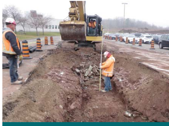
Figure 9.2.2: In this photograph, the contractor is verifying the depth of excavation while under supervision. (Source: CVC)
