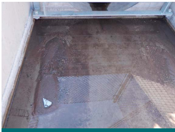
Figure 10.2.6: Along with measuring sediment depth in a proprietary stormwater treatment device, check the outlet structure (if accessible). If the device is functioning as intended this sedimentation should not be occurring, unlike this device. (Source: Aquafor Beech)
