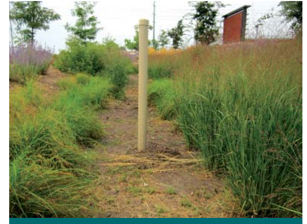
Figure 6.4.15: A plastic perforated standpipe is a simple, cost-effective, and low-maintenance overflow method. Starting the perforations at the desired elevation may meet surface storage requirements. (Source: Aquafor Beech)
