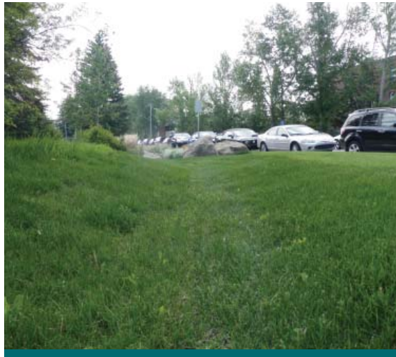
Figure 6.4.20: At the Marlowe Street retrofit project in the City of Calgary, grassed filter strips were used as a pre-treatment option between the inlet and bioretention area. (Source: Aquafor Beech)
