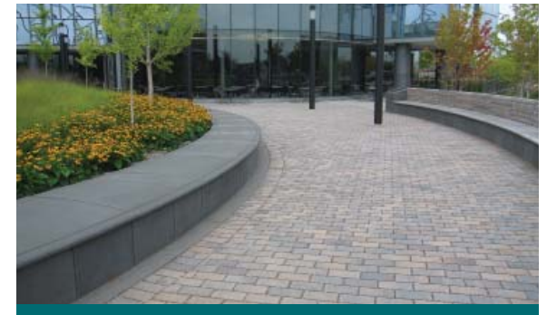
Figure 4.6.2: If your retrofit site includes a pathway from the parking lot to the main entrance, consider a retrofit using permeable pavement. Most permeable pavement meets accessibility standards and reduces the risk of slips and falls by preventing standing water and ice from forming on walking surfaces. (Source: CVC)
