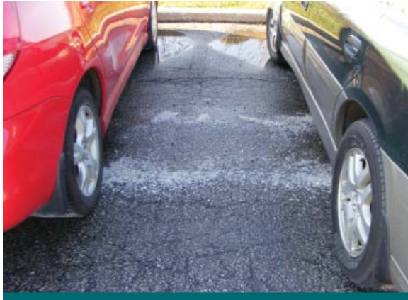
Figure 1.3.4: Over-applied de-icing salt to prevent slips and falls is common in many parking lots. Permeable pavements can reduce the need for salt. (Source: Aquafor Beech)
