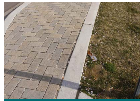
Figure 4.9.1: Further consideration of user behaviour may have resulted in a different LID solution for this location. This section of sidewalk is a preferred smoking location for the adjacent business and the cigarette butt waste stuck between the permeable pavers will be an ongoing maintenance problem. (Source: CVC)
