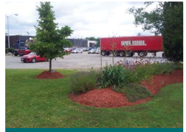
Figure 4.7.2: This landscaped area receives runoff from the adjacent staff parking lot, but not from loading bays. Bioretention is a suitable retrofit option in this area. (Source: Aquafor Beech)
