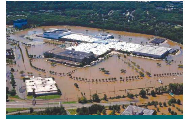
Figure 11.0.2: This shopping centre was forced to temporarily shut down due to significant urban flooding. In addition to lost business, flooding can result in the loss of goods. Improving drainage and reducing the amount of impervious surface could help alleviate urban flooding in this area. (Source: CVC)
