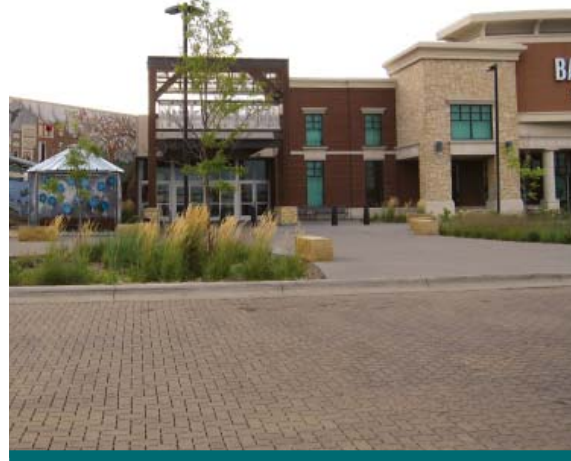
Figure 2.2.3: Permeable pavers come in a variety of shapes and sizes. They can be arranged in patterns that enhance site aesthetics. Here permeable pavers are used to mark a pedestrian crossing zone at a mall entrance. (Source: CVC)
