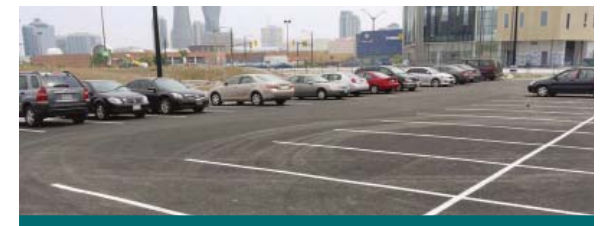
Figure 2.2.2: Porous asphalt can look quite similar to conventional asphalt. Site operators should track the location of permeable infrastructure to ensure that it is not paved over by future paving projects. (Source: CVC)
