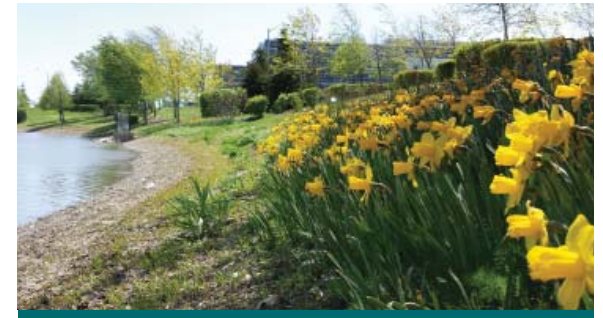
Figure 10.1.1: At this stormwater management facility, a municipal-private partnership approach to maintenance was established. The municipality is responsible for life-cycle activities that are critical to maintaining the facility, including outlet inspections and dredging. The land management company that owns the adjacent property is responsible for maintaining landscape features. (Source: CVC)
