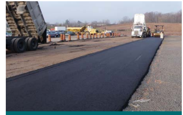
Figure 9.6.4: A temporary asphalt road used for construction access is one way to reduce onsite erosion caused by constant traffic from heavy vehicles and equipment. (Source: Aquafor Beech)
