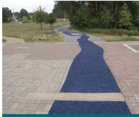
Figure 2.2.1: Pervious concrete can be dyed to suit site purposes. At this site permeable pavers are used in conjunction with coloured pervious concrete to produce a unique pattern on a pedestrian walkway. (Source: CVC)
