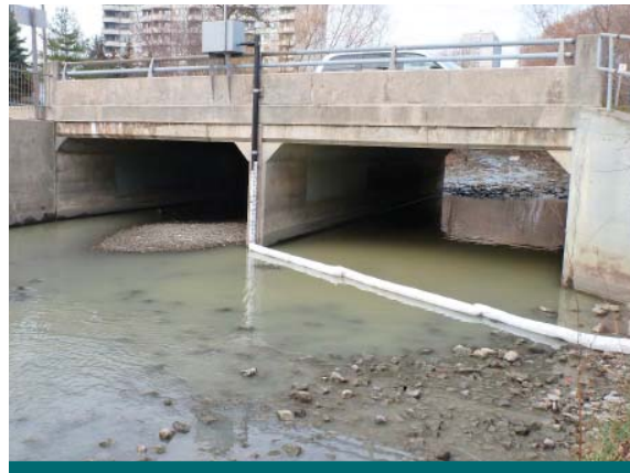
Figure 1.1.6: Spills entering water bodies can result in heavy fines for the polluter. This image shows a diesel spill in a creek. A filter sock was used to contain the spill. (Source: CVC)
