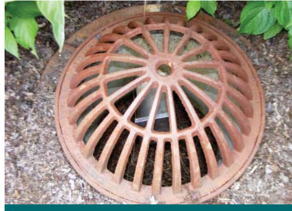
Figure 6.4.12: This metal atrium/dome overflow system is less susceptible to clogging than a flat grate. (Source: Aquafor Beech)
