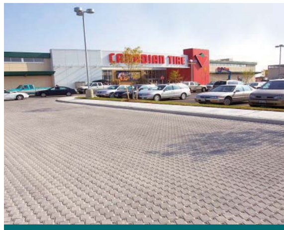
Figure 1.3.5: Canadian Tire can build its brand as a green corporation through the use of permeable pavement in its parking lot. (Source: Unilock)
