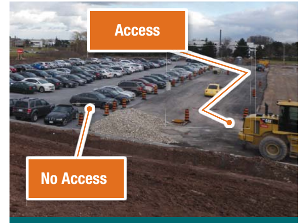
Figure 9.6.3: Consider site function during construction when planning a temporary asphalt road or any other erosion and sedimentation control. (Source: Aquafor Beech)
