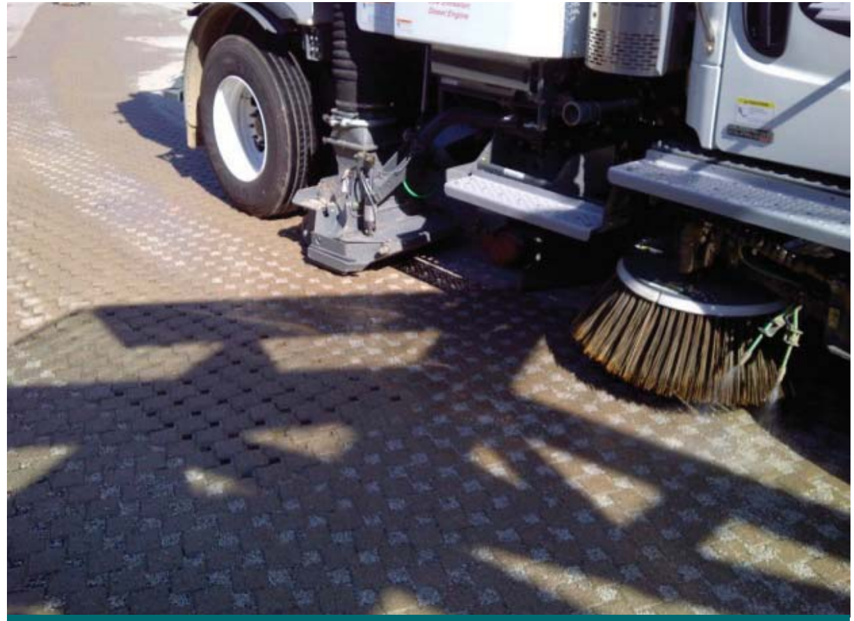
Figure 10.2.5: Vacuum sweepers will remove accumulated debris between block pavers, but can also remove aggregate from paver joints (note the voids behind the sweeper truck). Always replenish any lost joint aggregate following vacuum sweeping. (Source: Aquafor Beech)
