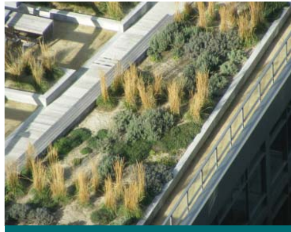
Figure 2.10.2: High-rise condominiums represent excellent opportunities for green roofs due to their large flat rooftops and the opportunity to create amenity space for residents. (Source: Aquafor Beech)
