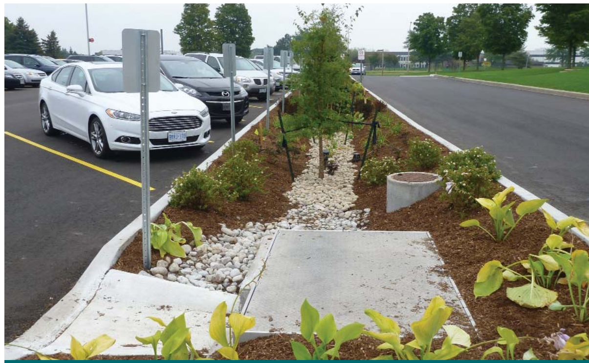
Figure 6.4.22: A Jellyfish® filter pre-treats stormwater within the bioretention area at the IMAX Project site. (Source: Aquafor Beech)
