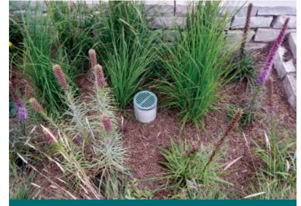
Figure 6.4.14: A plastic flat top overflow is cost-effective but susceptible to damage. (Source: Aquafor Beech)
