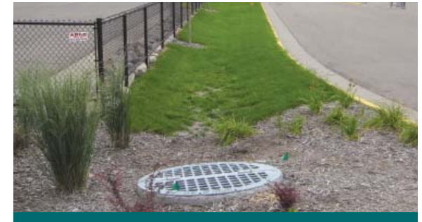
Figure 2.4.1: A long island separating an entranceway and parking lot is used to treat runoff with a bioswale. (Source: CVC)
