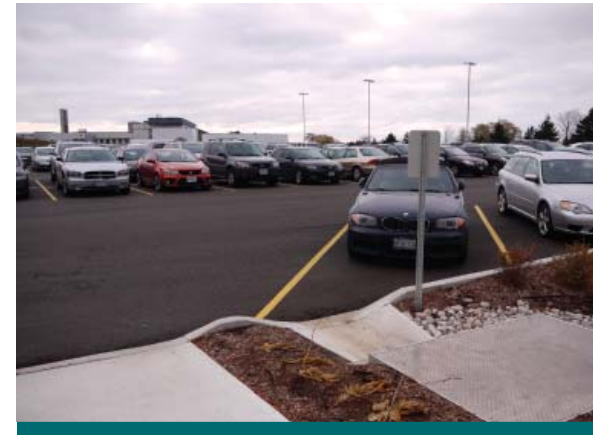
Figure 4.1.3: The layout of the site will determine the placement of practices on a site. Features like priority parking and wheelchair access can inform a retrofit design. (Source: CVC)
