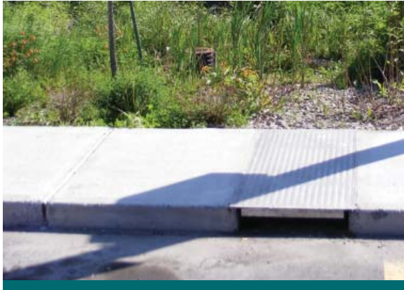
Figure 6.4.8: This grated curb cut is textured to prevent pedestrian slips. Grates should also be corrosion resistant. (Source: Aquafor Beech)
