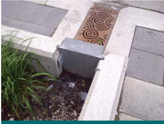
Figure 6.4.9: A gate has been added to this grated curb cut design to allow the facility to be closed during the winter. (Source: Aquafor Beech)
