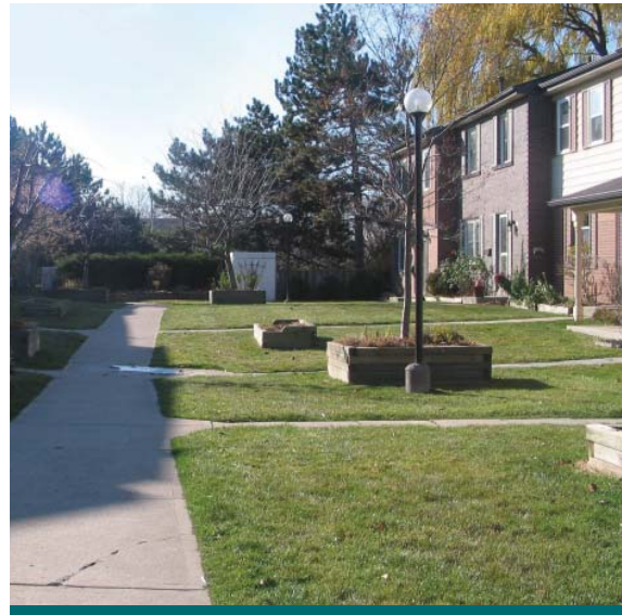
Figure 4.8.2: In many low-rise residential developments, a portion of the roof drainage is directed to conveyance features (ie. rear-yard catchbasins). In the Ganonoque townhouse complex in Mississauga, homes and common elements are built on top of the parking garage, extending the life of the parking lots. (Source: CVC)
