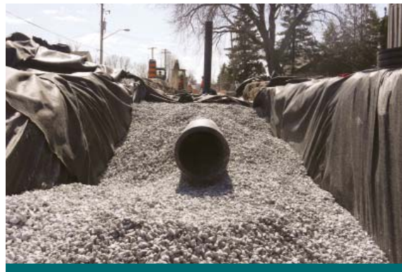
Figure 2.6.1: A perforated pipe is installed in a granular trench to encourage infiltration. (Source: Aquafor Beech)
