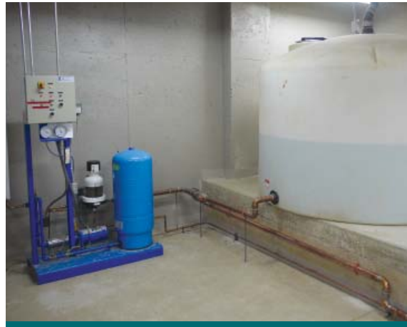
Figure 2.7.1: Rainwater can be stored in a variety of different locations, either outdoors or indoors. For instance, CVC's rainwater storage tank is located in the basement of its head office. (Source: CVC)
