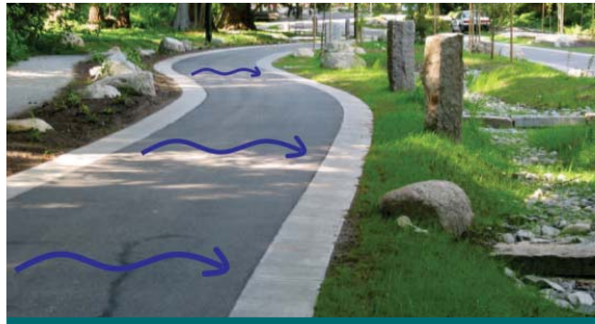
Figure 6.4.3: Flush curbs on both sides of this street allow for drainage from left to the bioswale on the right. (Source: City of Vancouver)
