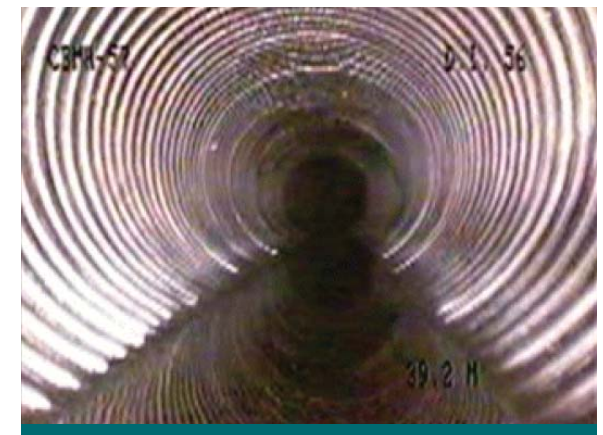
Figure 10.2.4: Video inspection (pipe scoping) is a rapid means of identifying issues with buried pipe. Look for indications of pipe collapse, blockages, or sediment buildup. This photograph from an Ottawa perforated pipe shows it to be in excellent condition even after more than 20 years of performance. (Source: City of Ottawa)
