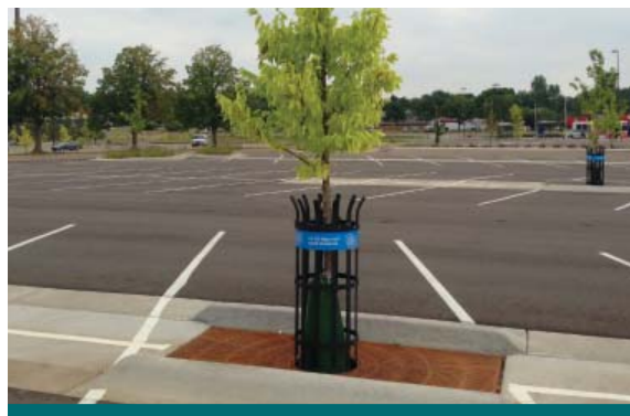
Figure 2.9.1: Precast tree planters can be used independently or as part of a treatment train with other LIDs to treat stormwater runoff. Here they are incorporated into a parking lot curb-and-gutter system. (Source: CVC)
