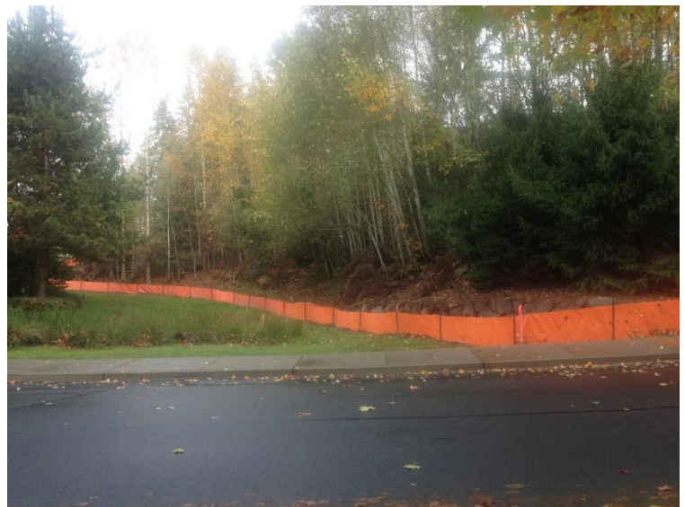
Figure 10. Silt fencing at construction site.
