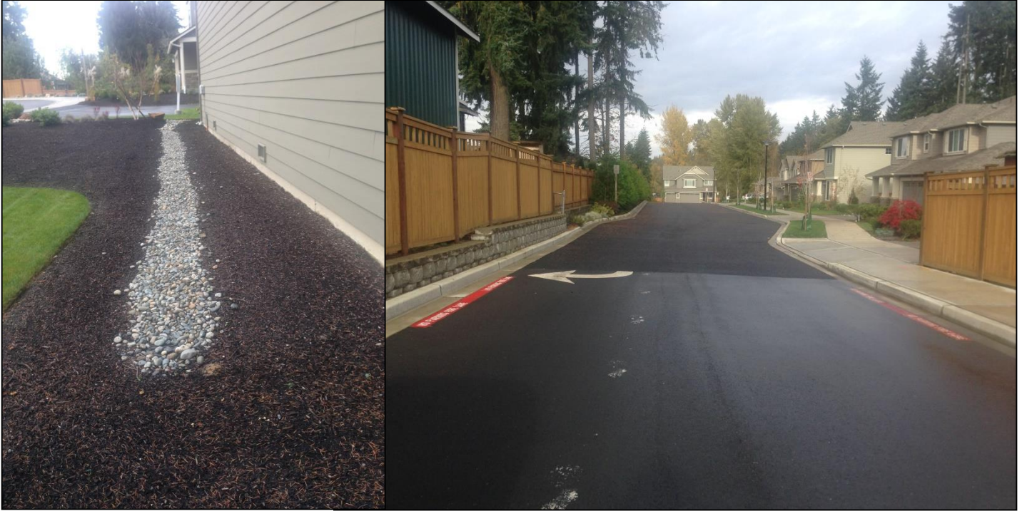
Figure 9. New development with a large suite of LID/GSI techniques including infiltration and permeable pavement (along with conventional pavement).
