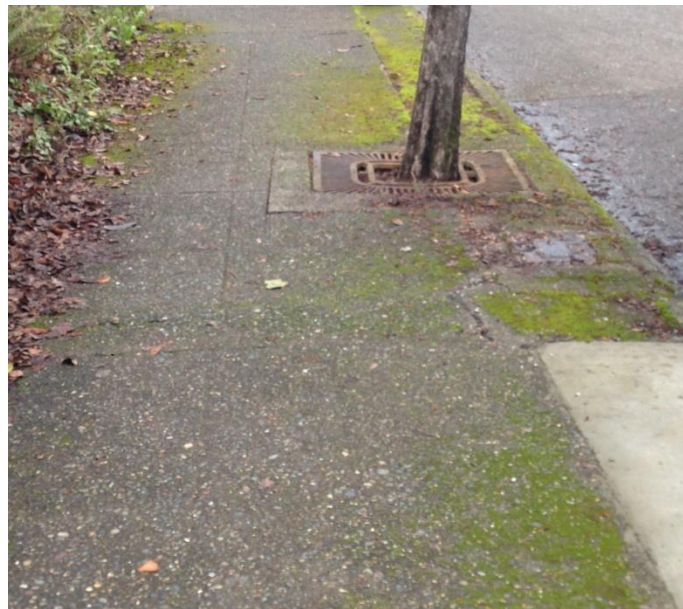
Figure 6. Top photos: Moss on permeable pavement sidewalks showing contrast with regular pavement. Bottom photo: Moss on regular (aged) pavement sidewalk. Photo credit for top right photo: Ross Freeman, City of Mercer Island.
