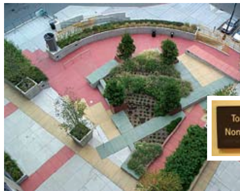
Clockwise from top: King County stores roof runoff in cisterns at the King Street Center in Seattle, uses it to flush bathroom fixtures and irrigate landscaping.
