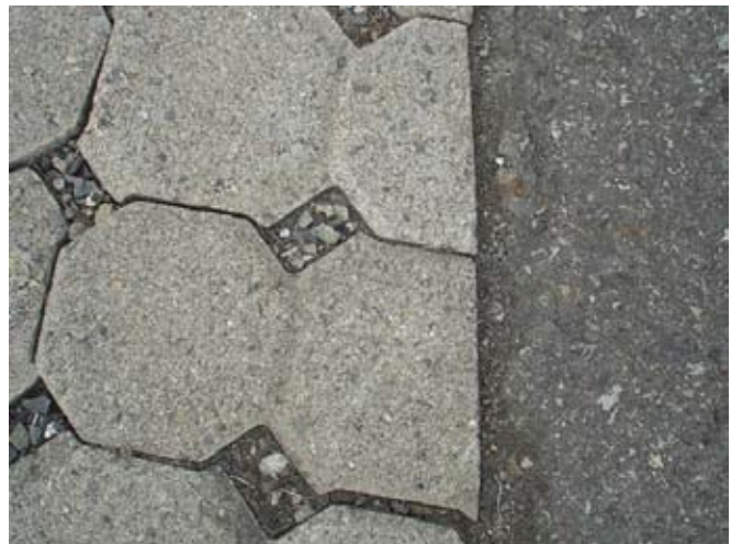
Permeable pavers are used to retrofit a Park & Ride.
