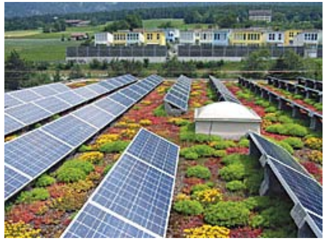
Vegetated roofs can be used in conjunction with solar power, a green building technology that has a quick return on investment.
