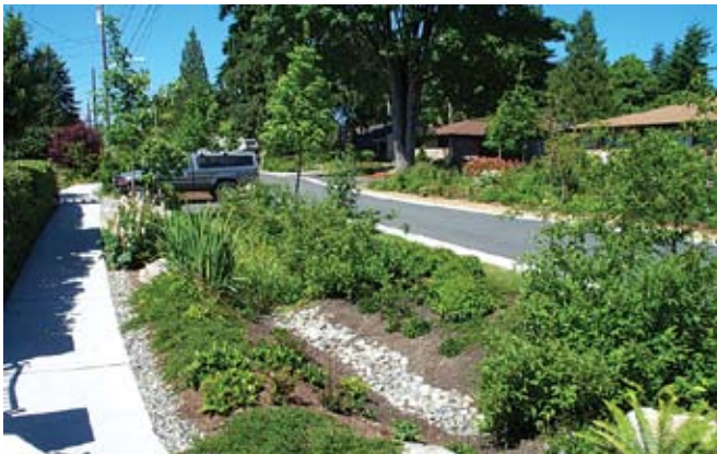
Conveyance swales in a Seattle Public Utilities project are 98% effective at storing and absorbing wet season runoff.
