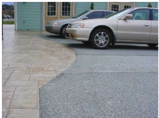
Porous concrete can be used for aesthetically pleasing & functional parking areas.
