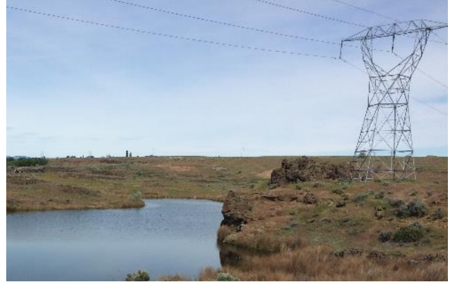
Powerlines in Grant County
