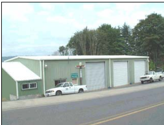
City of Kalama, Public Works Shop
