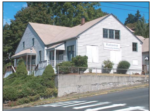
Kalama Community Building
