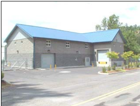
City drinking water treatment facility
