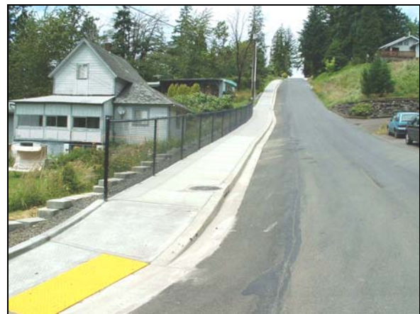
Sidewalk improvements along Fifth Street
