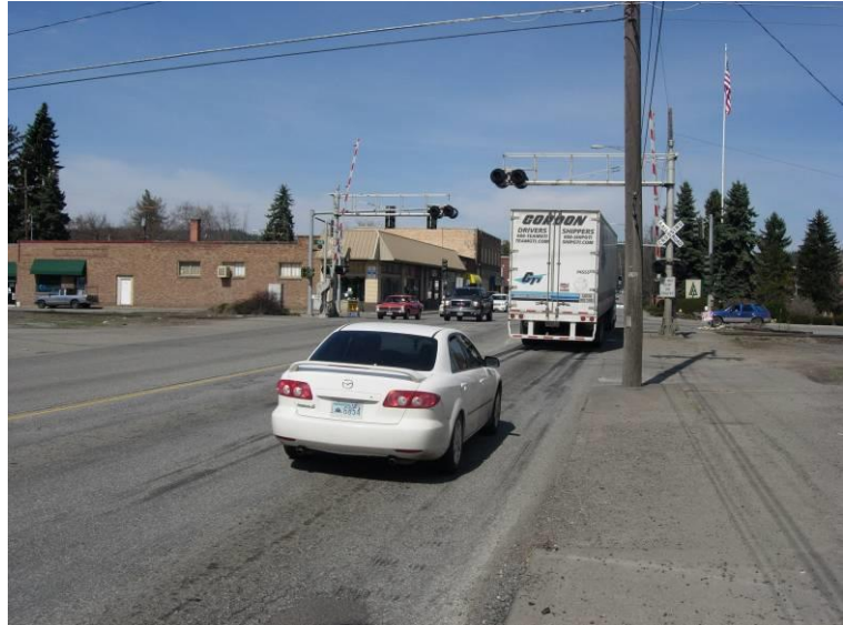
Figure 7 – The Argonne corridor has many cross streets, a railroad crossing and a business center. Photo: City of Millwood
