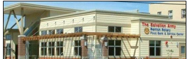
The Salvation Army Services Center, Credit: City of Renton
