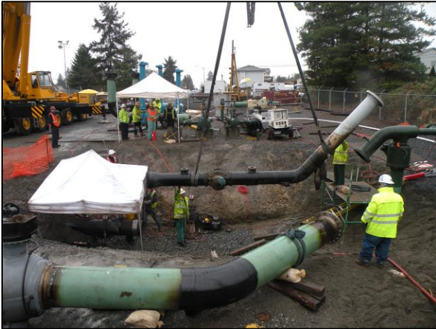
Natural Gas pipe replacement, Credit: PSE
