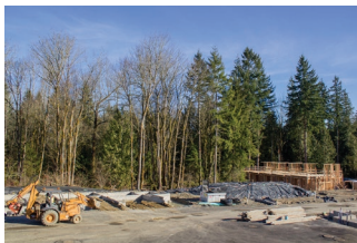
New housing development under construction
