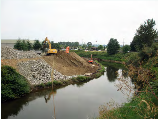
Levee repair at Lilly Point
