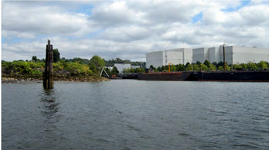
Tukwila's Manufacturing/Industrial Center is an important regional industrial center located along the Duwamish River.
