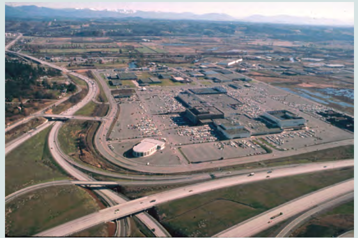
I-5 / I-405 Interchange – February 1973
