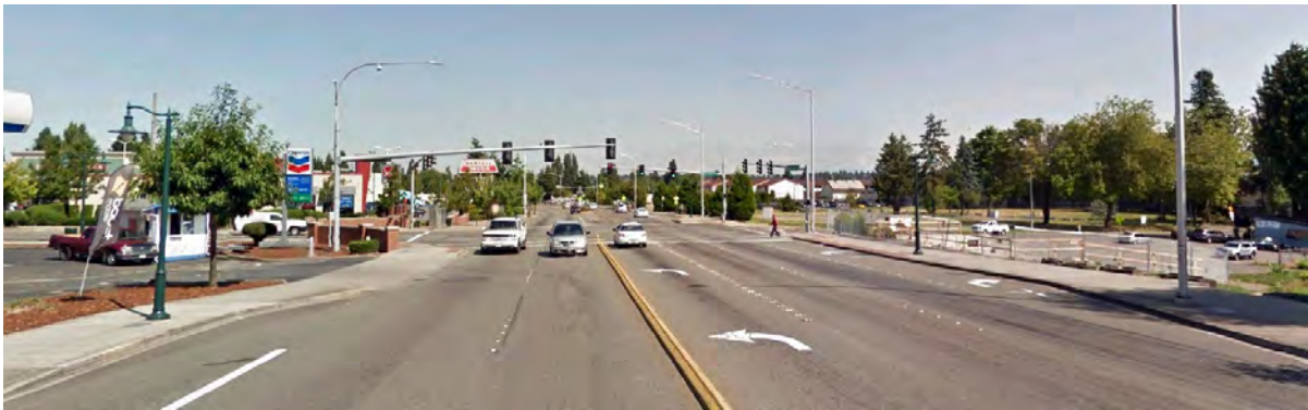
Figure 2. Looking north on TIB towards the intersection with S. 144th Street (2015)
