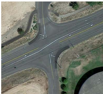
Raised Median on Hwy 12 creates a barrier for north-south travel
