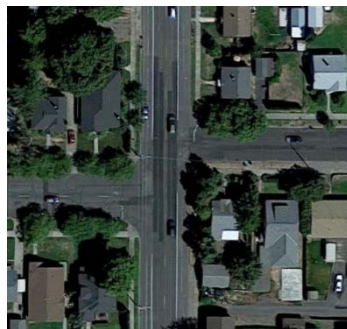
Off-set intersection of Howard St/Chestnut St limits east-west travel and serves as system deficiency
