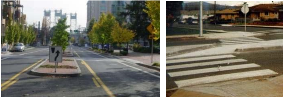
Figure 9: Example Center Medians with Pedestrian Refuge Islands
