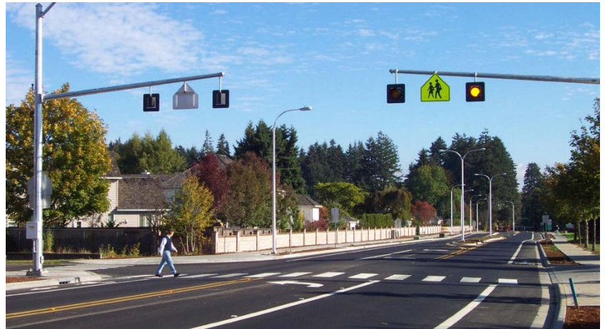
Figure 13: Example overhead flashing beacon
