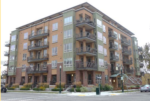
Apartment buildings with stoops and both vertical and horizontal articulation
